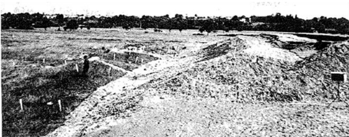
Figure 3. 37 View of the Cubzac embankment after failure (L A Rochelle et al. 1982)
