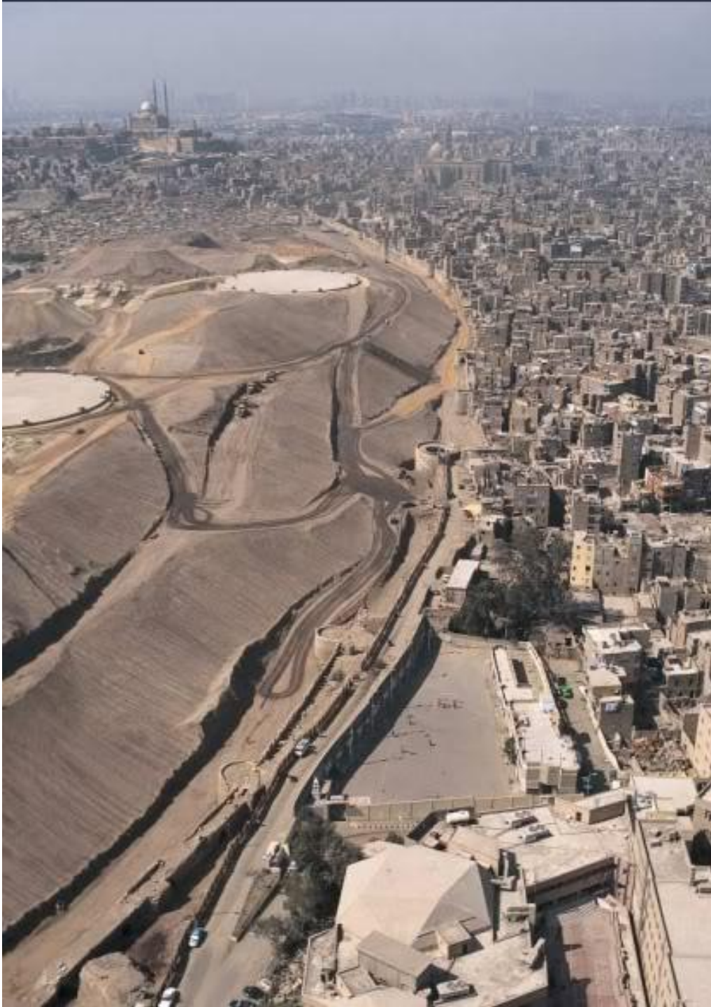
Figure 3.17: Al Azhar Park site under grading and construction, retrieved via www.akdn.org
