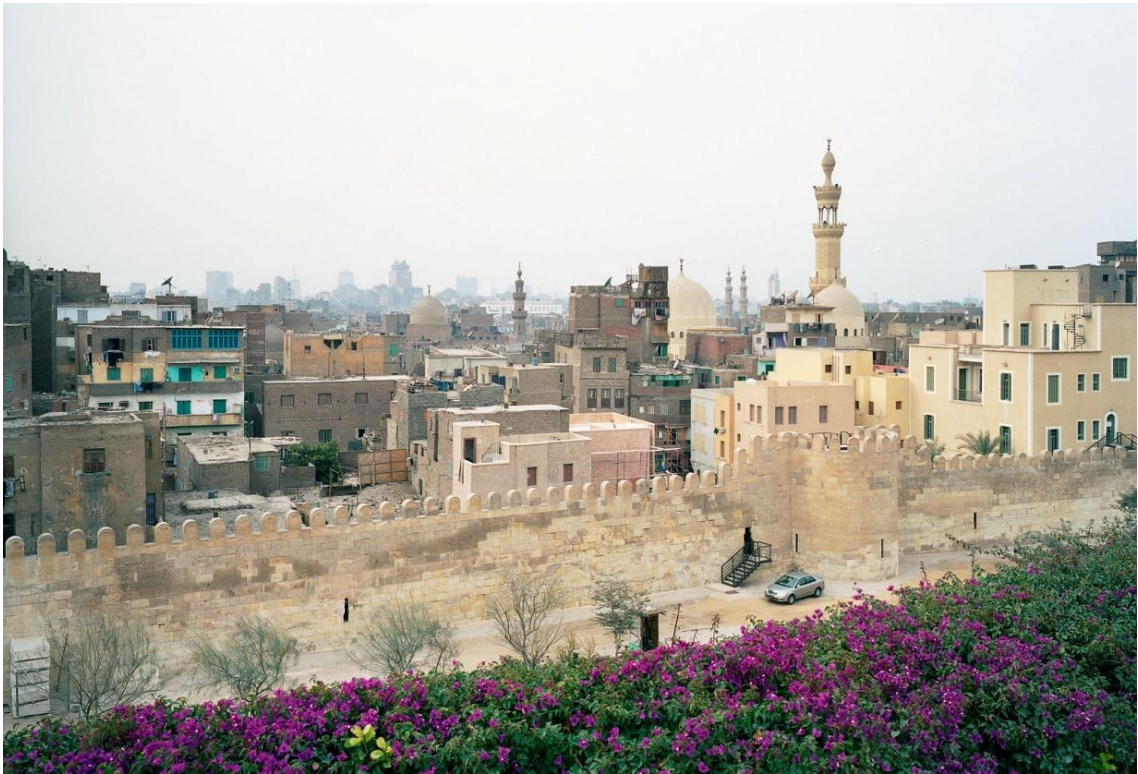
Figure 3.19: The restored 12 th century Ayyubid wall, separating the park from Darb el Ahmar neighborhood, retrieved via www.wikipedia.org/wiki/Al-Azhar_Park
