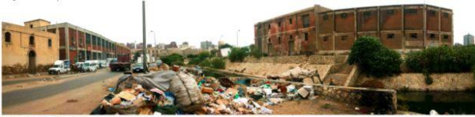
Mina el Bassal suffers from complete abandonment
