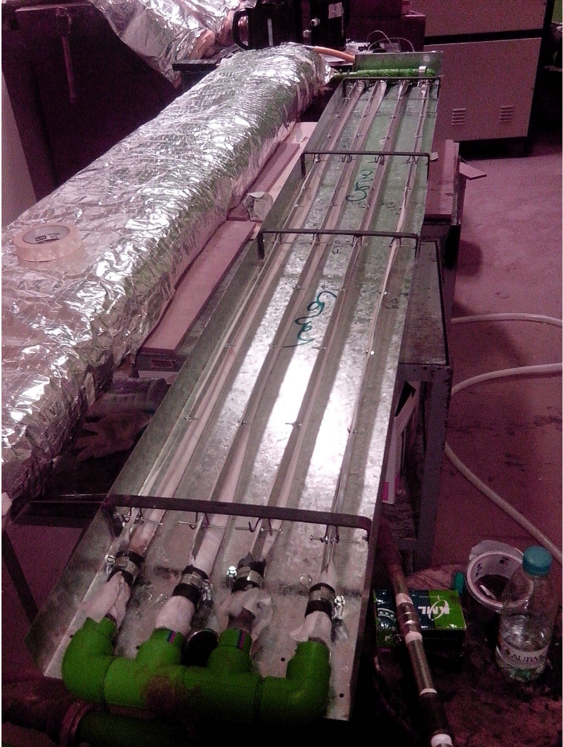
Figure 19: Permeable pipes assembled in the dehumidifier
