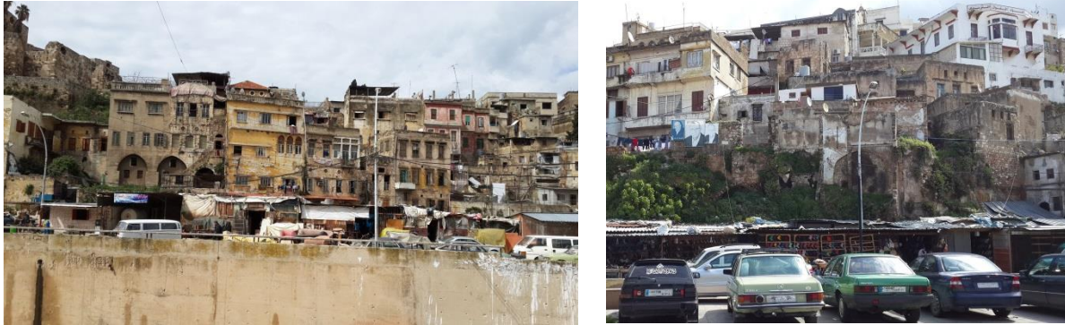
Figure63 : Buildings along the Abu Ali River
