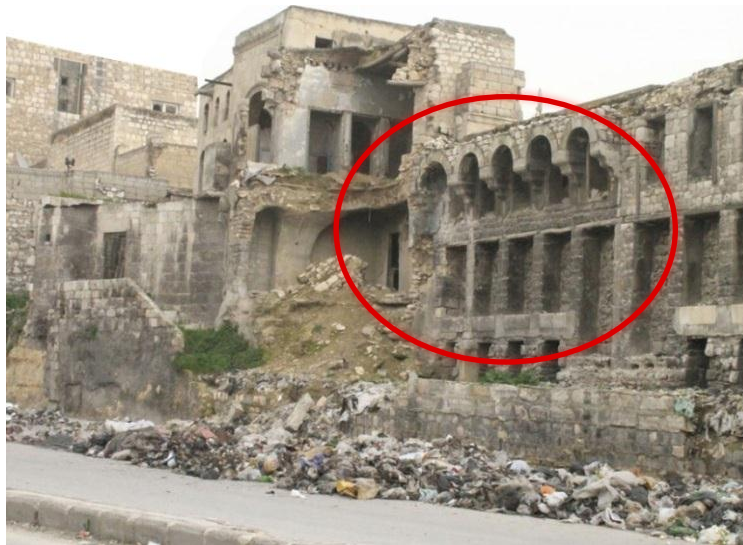
Figure 101. Image showing the bisected façade on the edge of the boulevard
