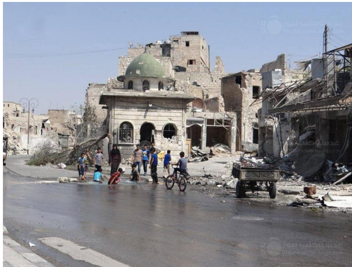
Figure 68. Image showing the destruction of the buildings in Qadi Askar boulevard area because of the war
