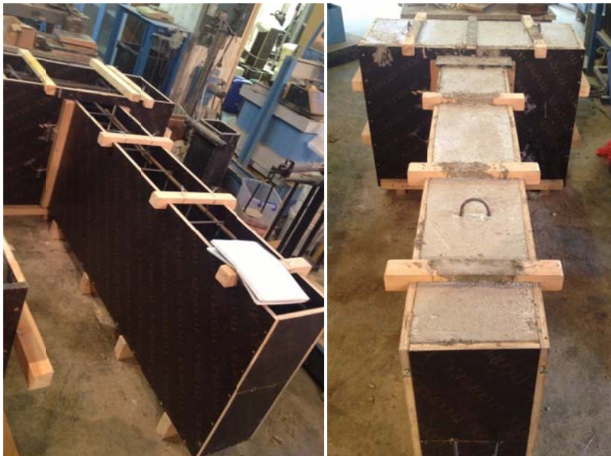
Figure 7. Formwork with top wooden braces before and after casting
