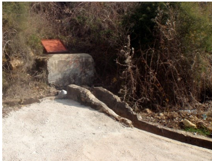
Figure 27 Irrigation canal pumping station
