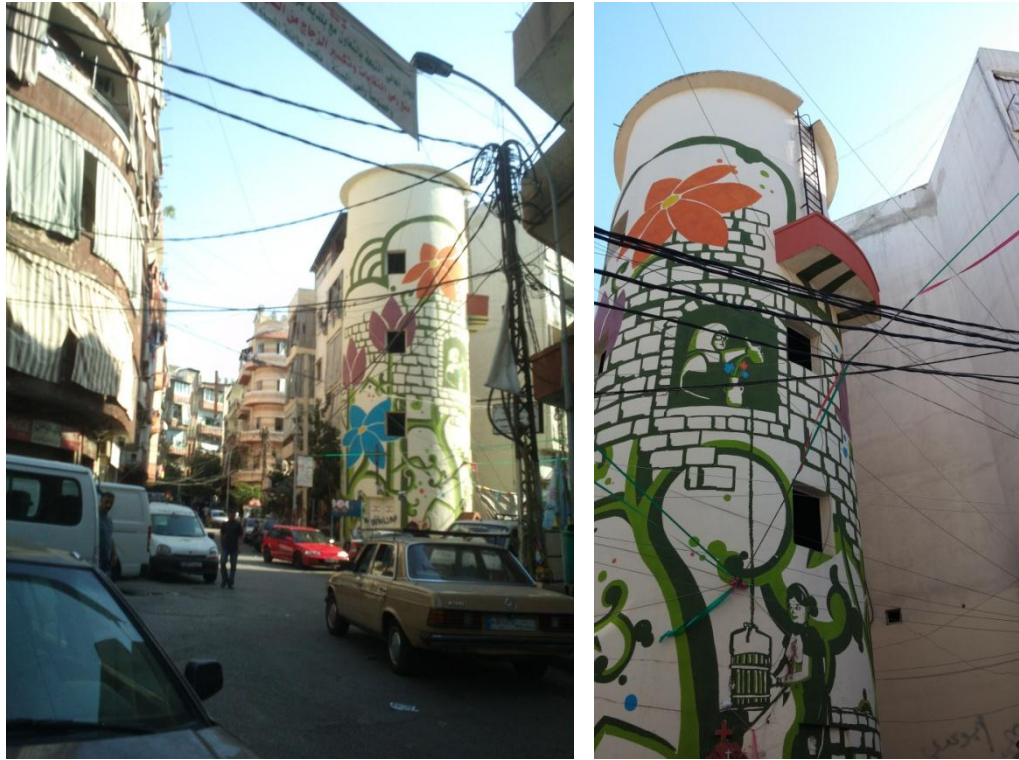
Figure 30: Water tower (حاووز)
