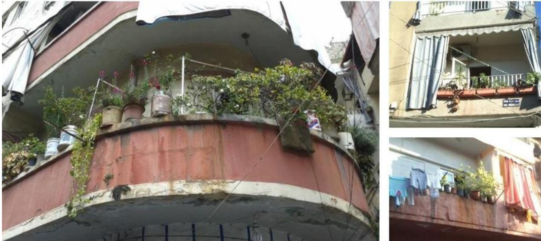
Figure 74: Nabaa's green balconies
