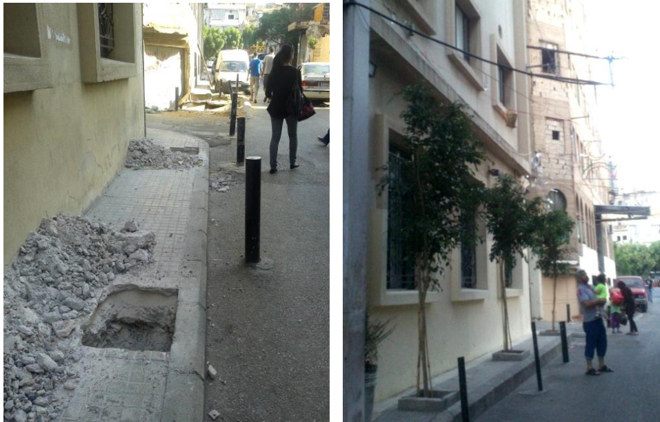
Figure 81: A narrow sidewalk before and after planting ornamental Ficus trees.
