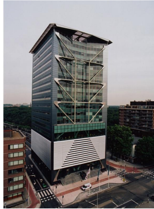
Figure 3.20: Maleitoren Building (Source:vno-new)
