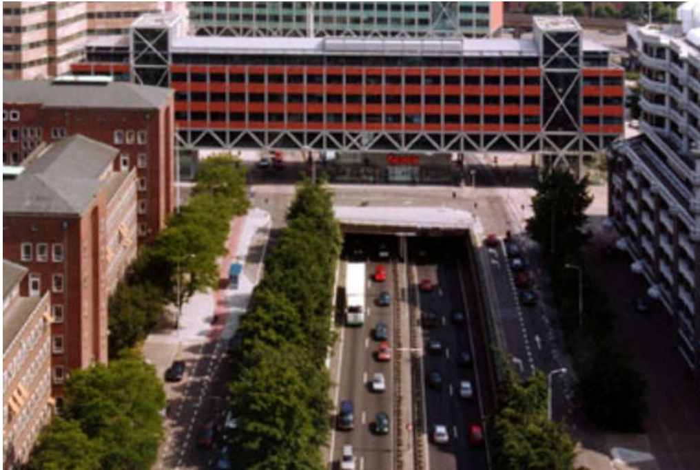
Figure 3.22: Equinox Building (Source:zja)
