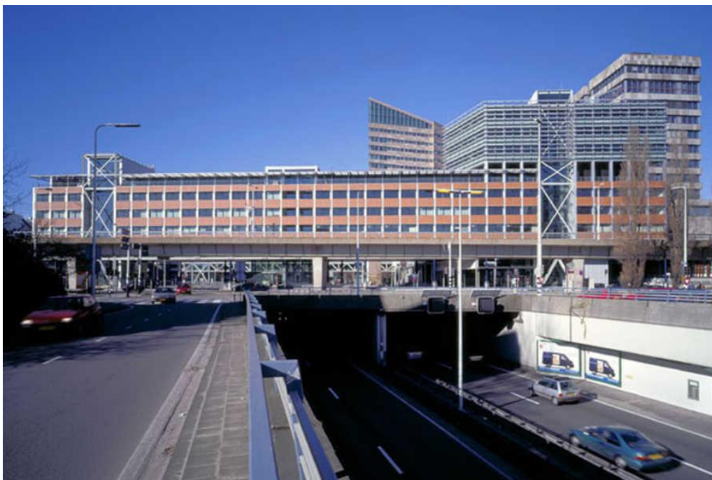
Figure 3.22: Equinox Building (Source:zja)
