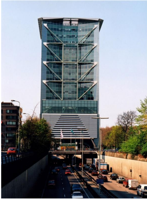
Figure 3.19: Maleitoren Building (Source:vno-new)
