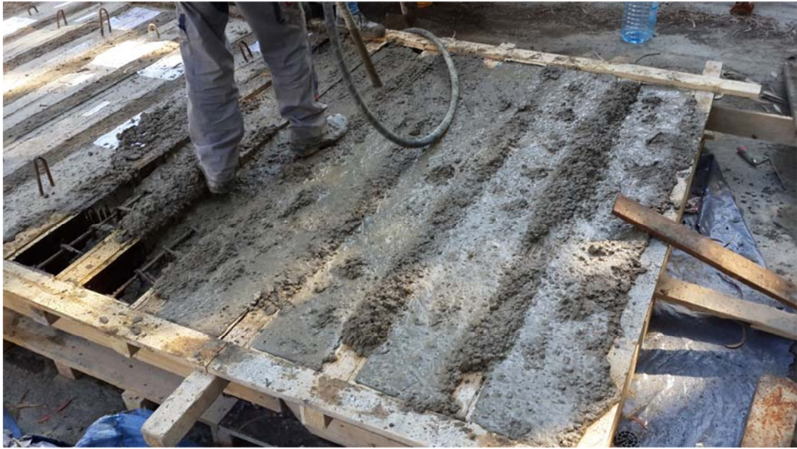
Figure 8-15: Concrete consolidation by vibrator
