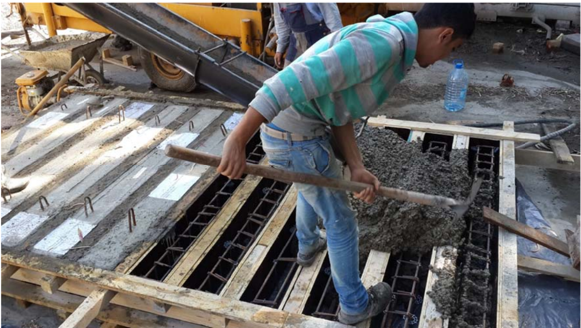
Figure 8-13: Concrete pouring
