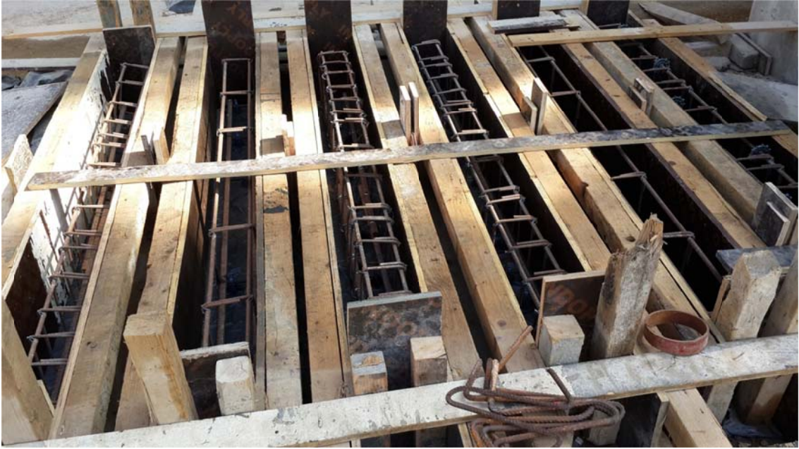
Figure 8-5: Assembled Formwork for set of six beams
