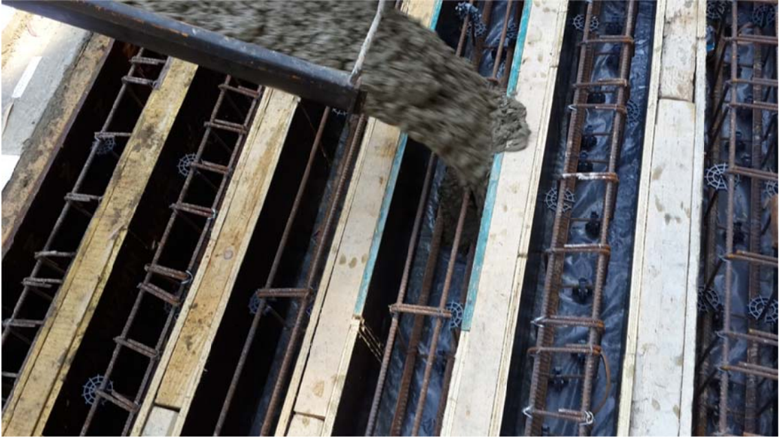
Figure 8-13: Concrete pouring
