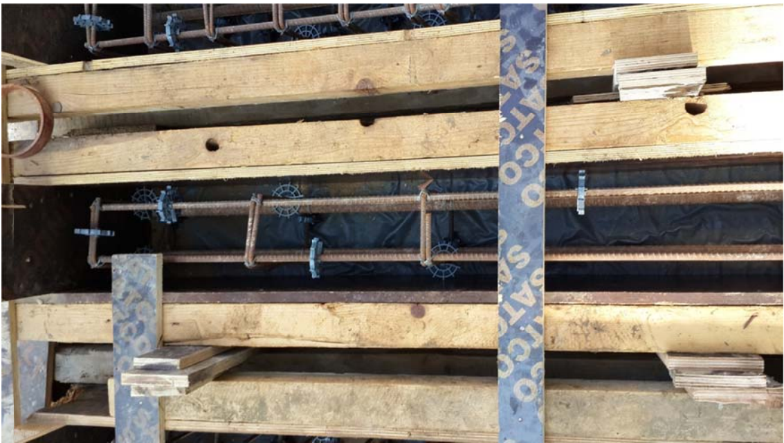
Figure 8-5: Assembled Formwork for set of six beams
