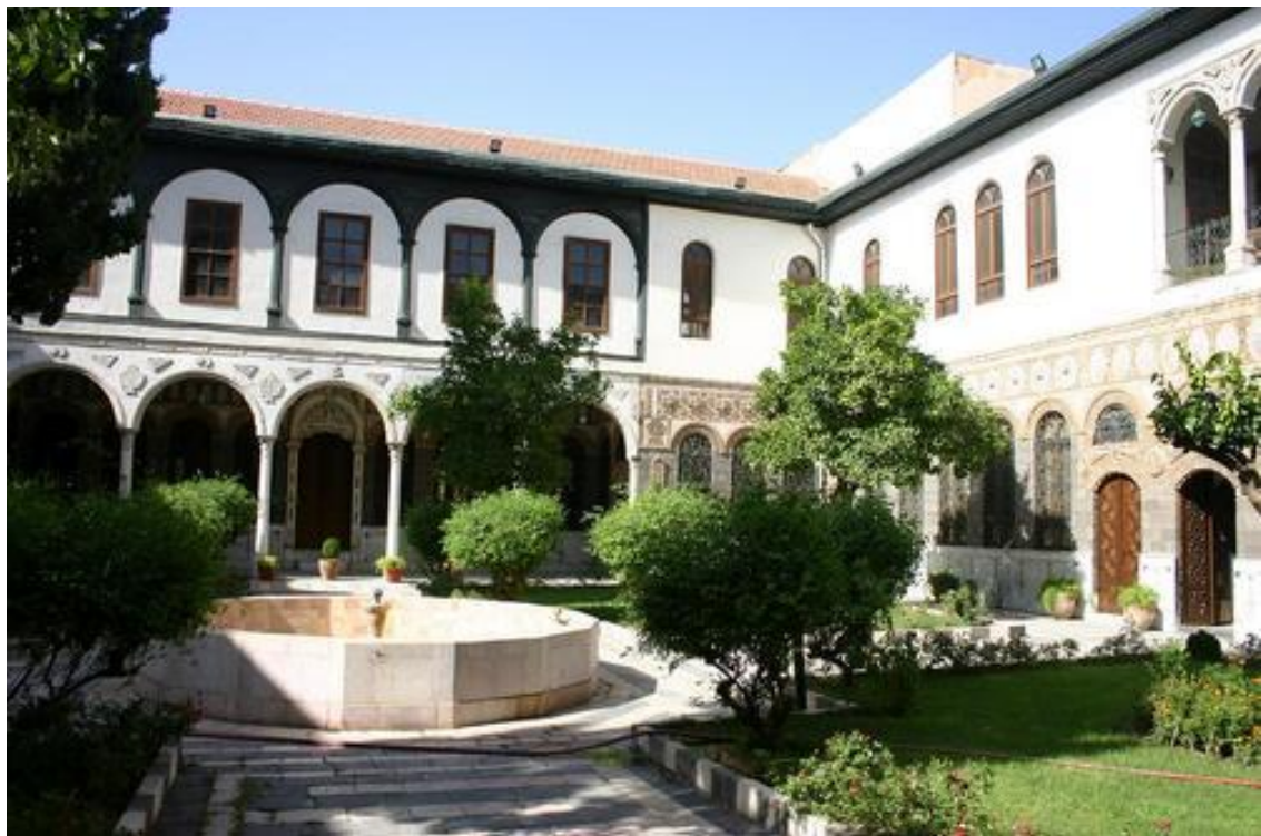
Figure 4.9: A photo shows the Damascene house's courtyard (Google.com1. 2015)
