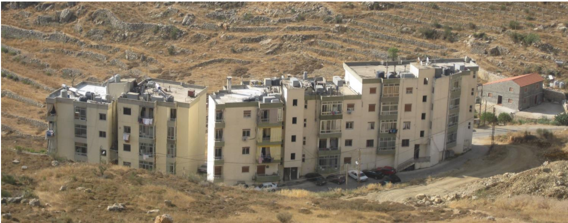
Figure 54. Jezzine fabric .This photo illustrates the new fabric in Jezzine West side. Photo was taken by Neaimeh, R.2015.
