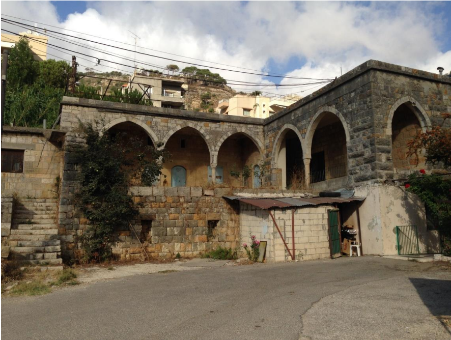
Figure 40. Jezzine fabric .This photo illustrates a gallery house in Jezzine core. Photo taken by Neaimeh, R.2015.
