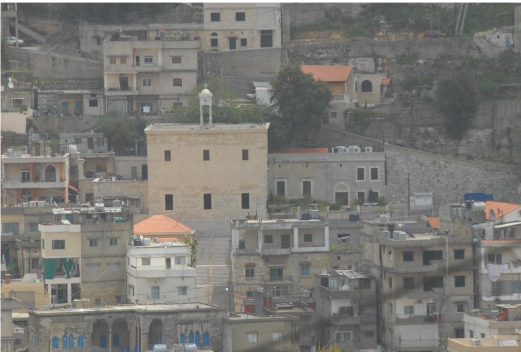
Figure 97. Jezzine Mar.Maroun Church, stairs and surroundings area. This photo illustrates, the core area in Jezzine, that plays a central role in the collective memory of people in the area: Photo Taken by Rahal,G.2015.
