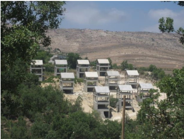
Figure 2. New developments in Jezzine town, taken by Author 2016.
