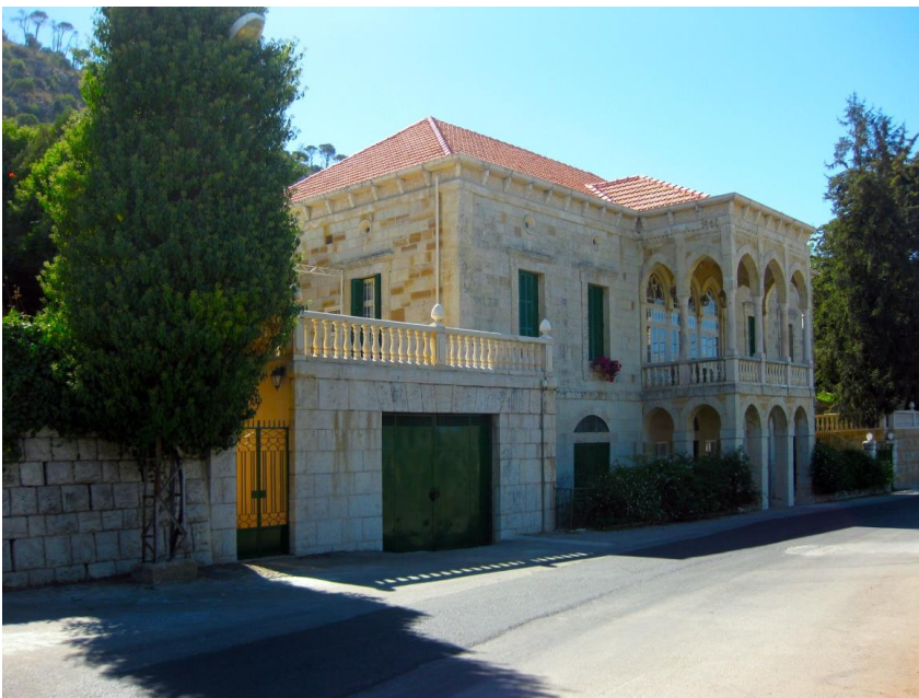
Figure 39. Jezzine fabric .This photo illustrates a triple arches house in Jezzine core. Photo taken by Neaimeh, R.2015
