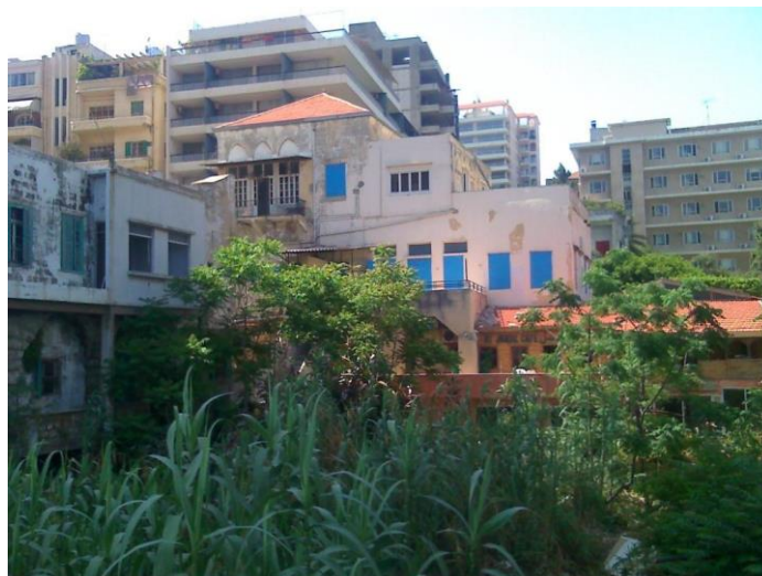
Figure 41: The previous Jamal and Normandy Beach after backfilling of the port (Source: Atallah)
