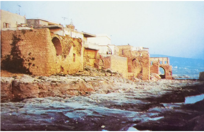
photograph of the old coastal houses before renovation
