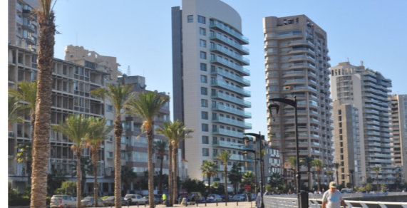
High Rise Residential Buildings
