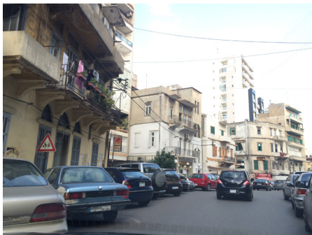
buildings mixed with residential and commercial uses
