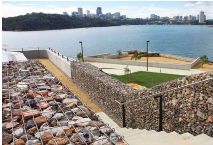
Figure 7: recycled gabion wall
