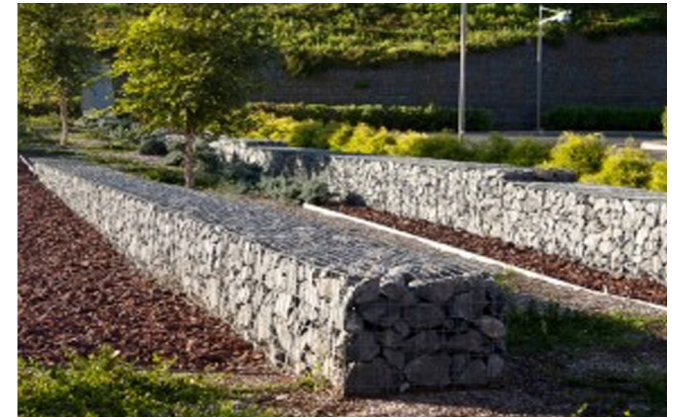
Figure 25: recycled gabion wall
