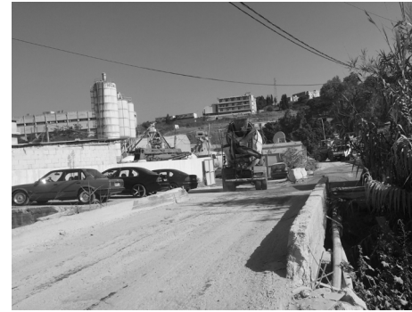
Figure 102 : road to river
