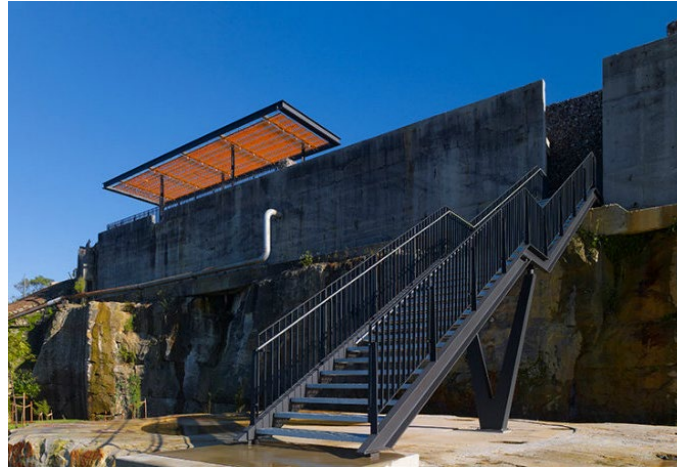
Figure 4: working with existing topography
