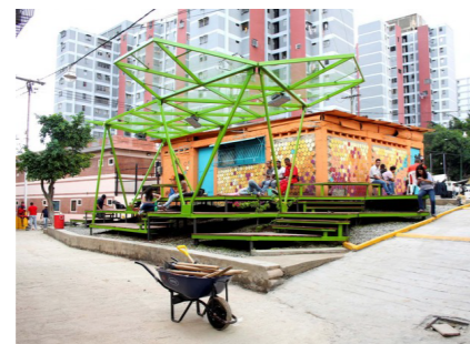
Fig. 6 After Intervention / Side View
