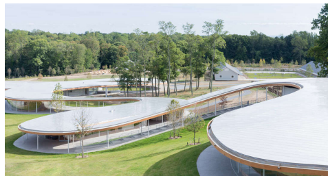
Case Study: The river building
