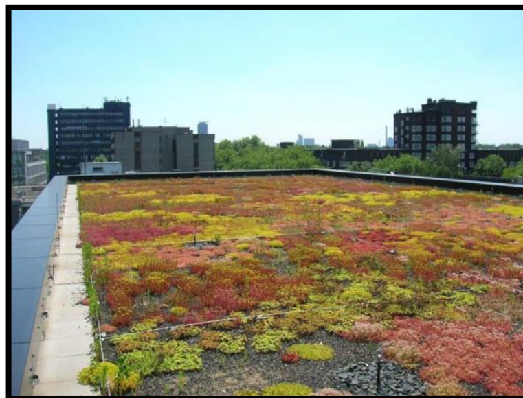
Figure 4 Extensive green roof (Source: www.greenroofs.com )
