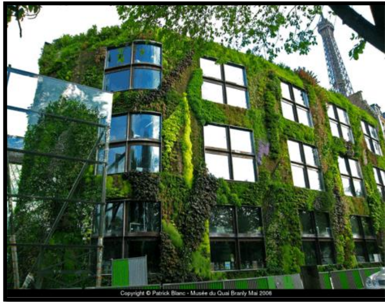
Figure 6 A living green wall (Source: http://www.greenroofs.com/ )
