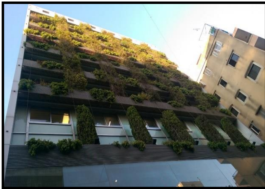
Figure 41 Existing building with a green facade and dangling vegetation
