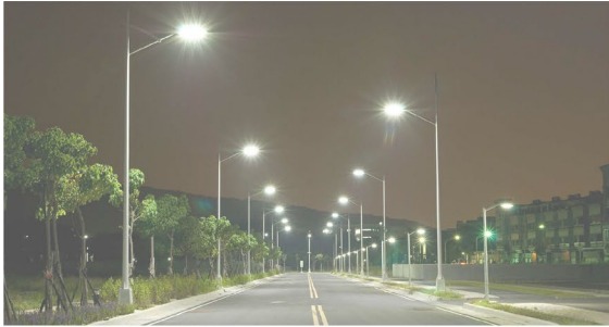
Lighting of the main road
