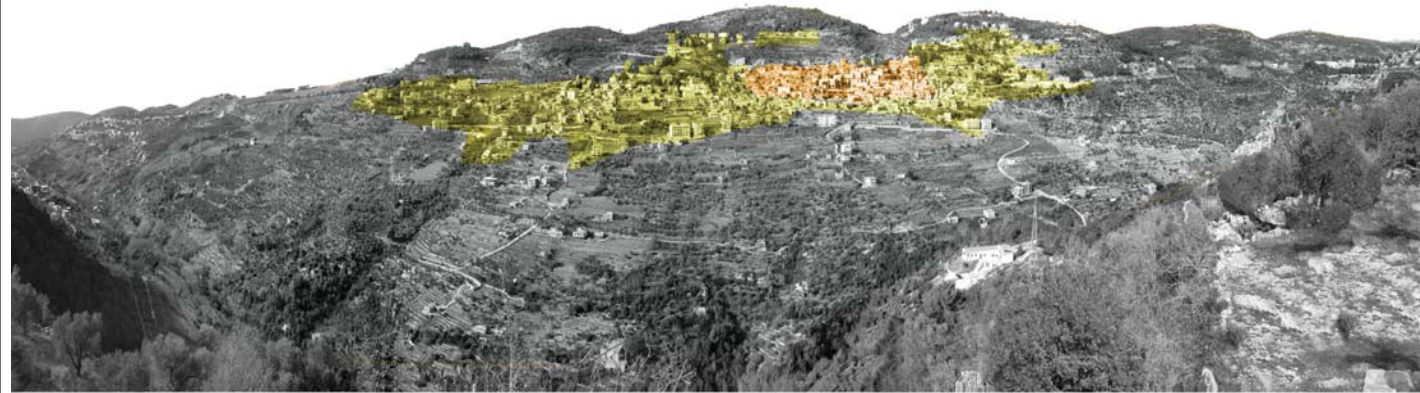
● URBANIZED LAND ● HISTORICAL ZONE FIG 10: PERSPECTIVE SHOWING URBANIZED ZONE IN DEIR EL QAMAR
