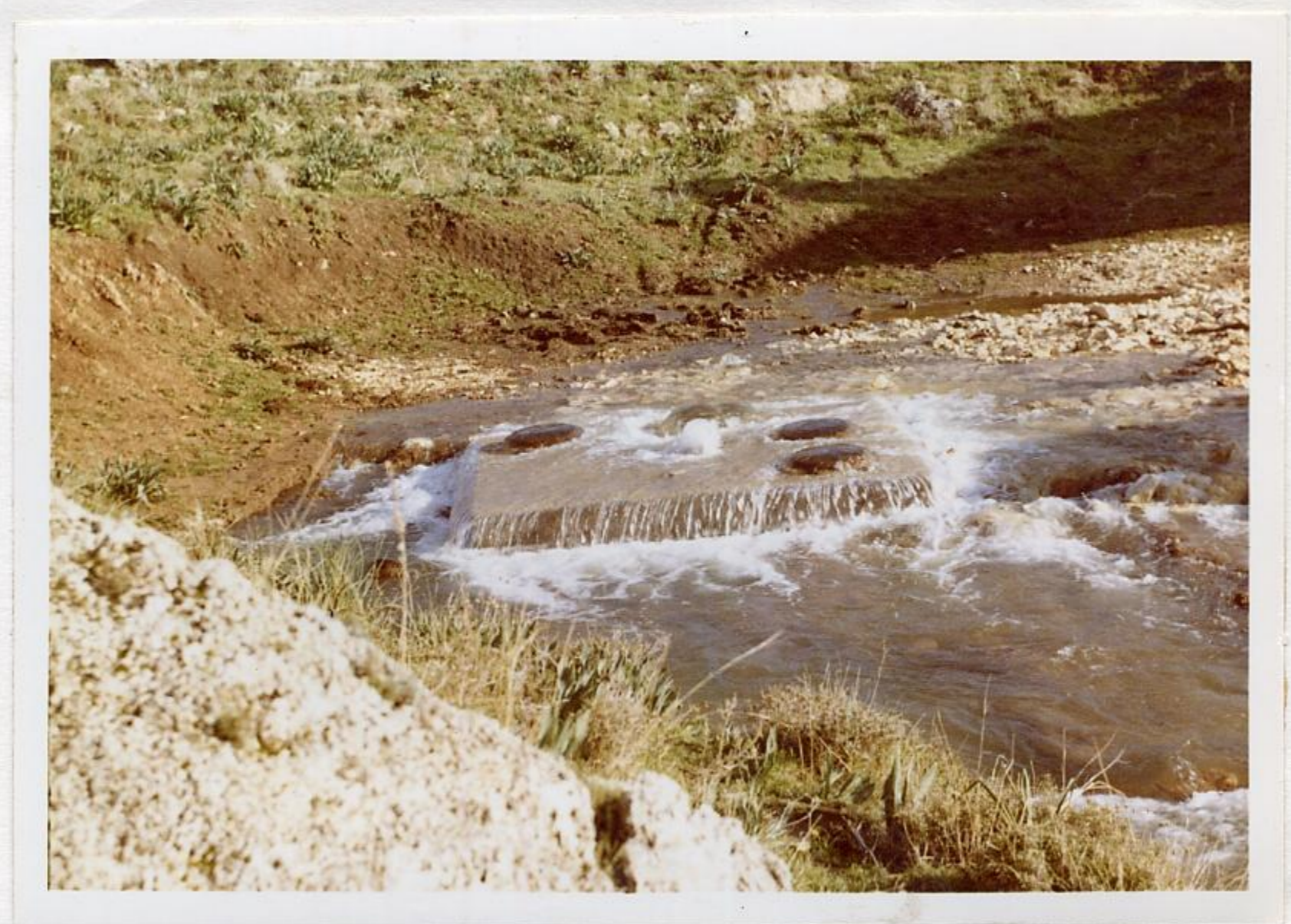
Photo 15-Artesian flow in Sink-hole "C". Concrete slab with wells 50, 51, 52, 53.
