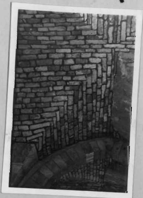
Photo N° 30 example of uncoursed latest Crusaders masonry.
