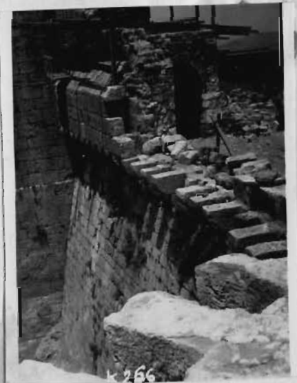
Photo N° 21 showing arab corbellement used as defence; note the difference with the previous one.
