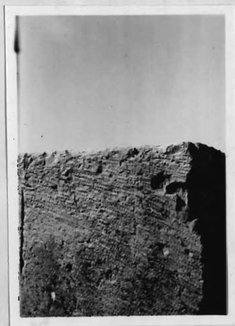
Photo N° 24 and 25 showing teeth edge dressed stones of Crusaders peroid, note the difference in the width of teeth.
