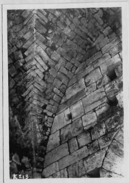
Photo N° 1 and 2 showing the solutions given to the goined arch corners.
