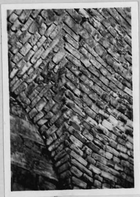
Photo N° 1 and 2 showing the solutions given to the goined arch corners.
