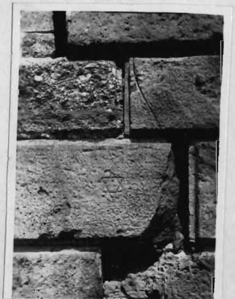
photo N° 9 and 10 showing crusader form of drafted stones and a mason mark.
