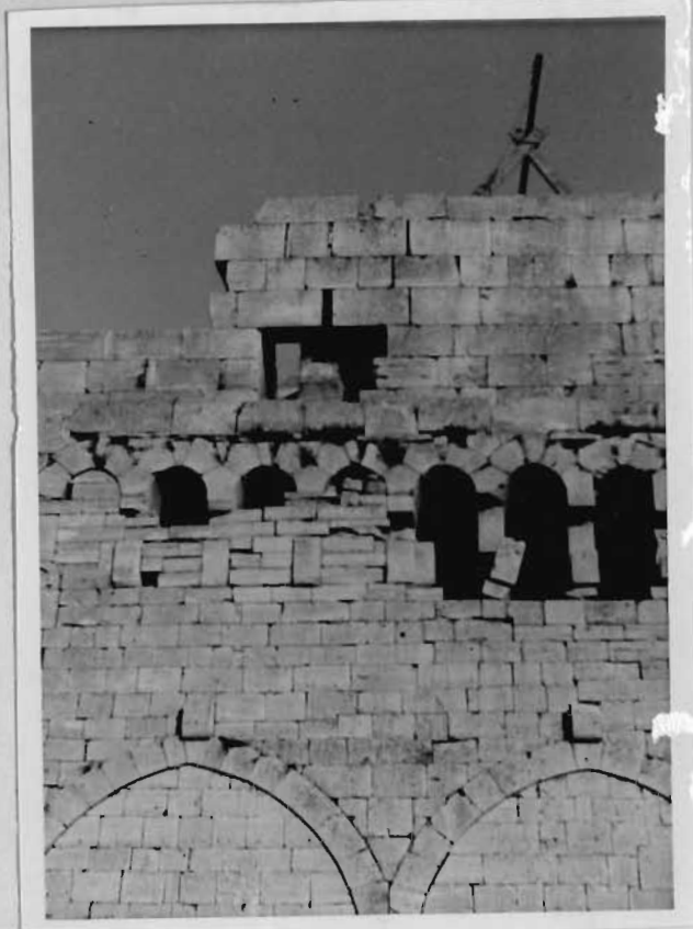
Photo 19 showing the double W.C.s of Tower P Crac protruding stones on the top of the arcs are the tie stones between two walls.
