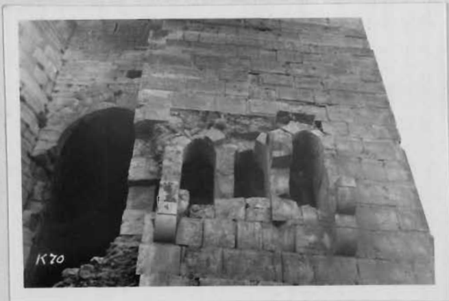
Photo N° 20 showing crasaders corbellement used as W.C. and and construction of drafted and smooth stone.
