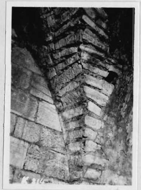
photo 11, 12, 13, and 14 showing second period early vault and goined corners.
