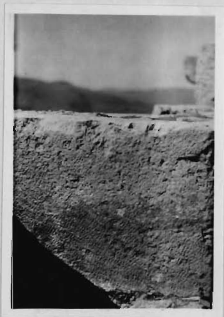
Photo N° 24 and 25 showing teeth edge dressed stones of Crusaders peroid, note the difference in the width of teeth.
