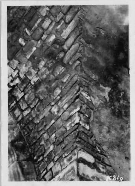
photo 11, 12, 13, and 14 showing second period early vault and goined corners.
