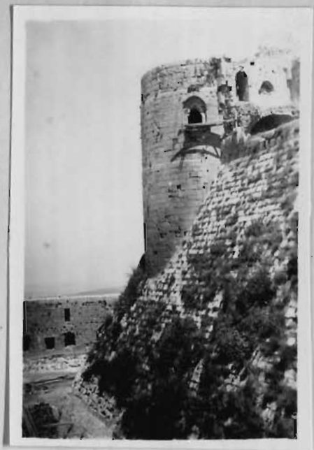
Photo N° 29 example of battered wall early second period.
