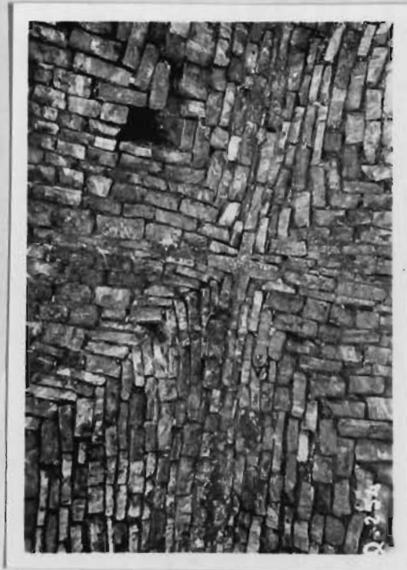
Photo 5 and 6 showing goined corner and top point solution First peroid "B"
