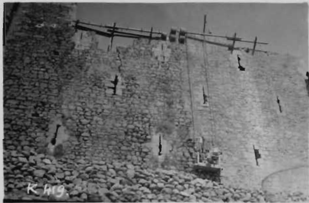
Photo N° 30 example of uncoursed latest Crusaders masonry.
