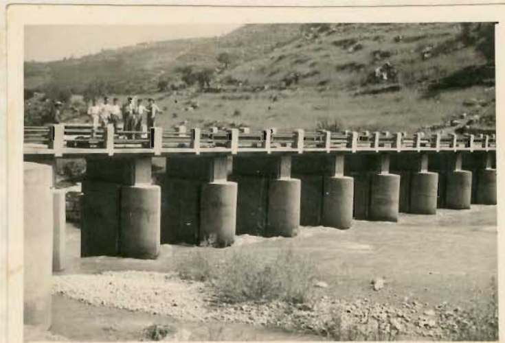
The same headworks seen from upstream.
