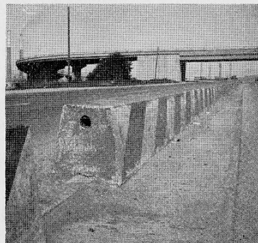
Figure No. 6 Concrete median barrier
