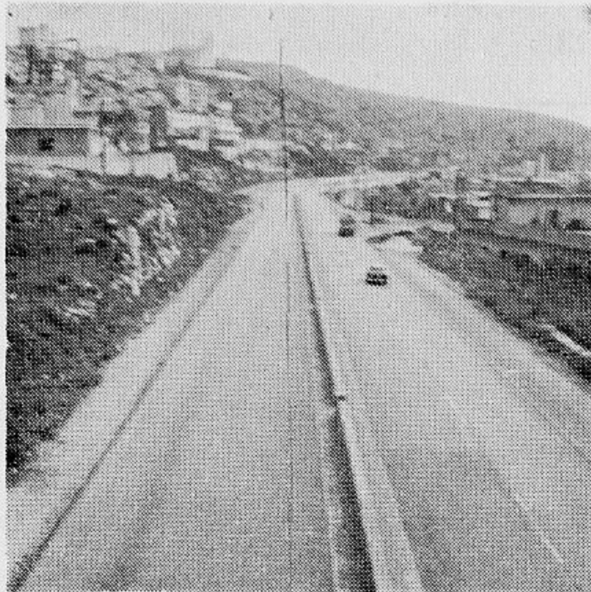
Figure No. 10 Concrete median barrier - type B - Location under study
