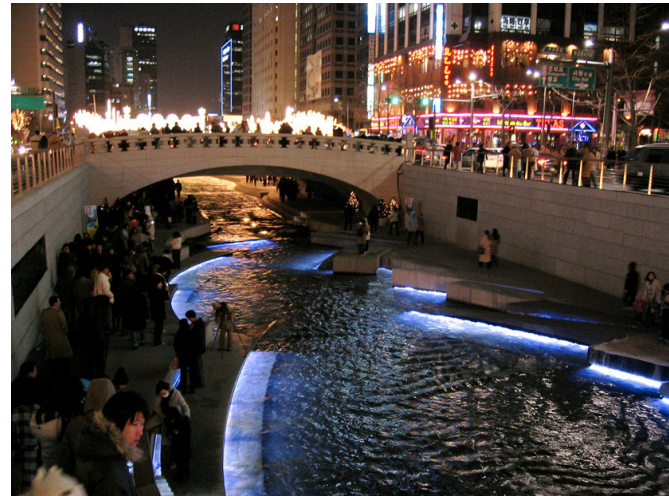
Underwater lighting - crossing bridge
