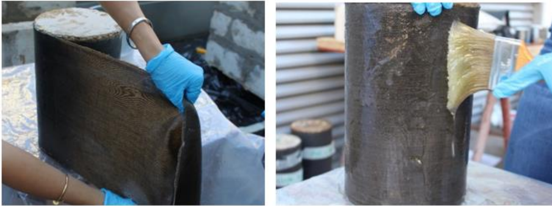
Figure 20. Application of hemp FRP wraps.
