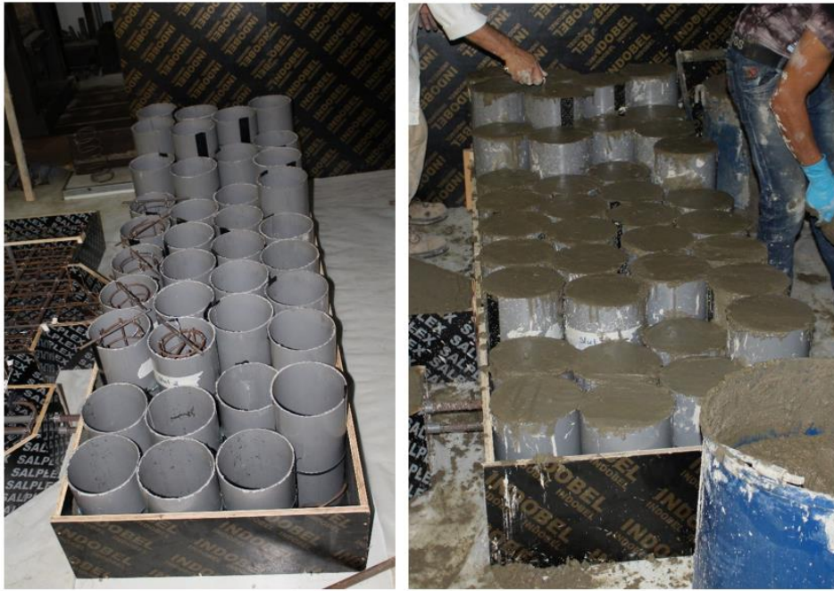
Figure 18. Casting of concrete columns.
