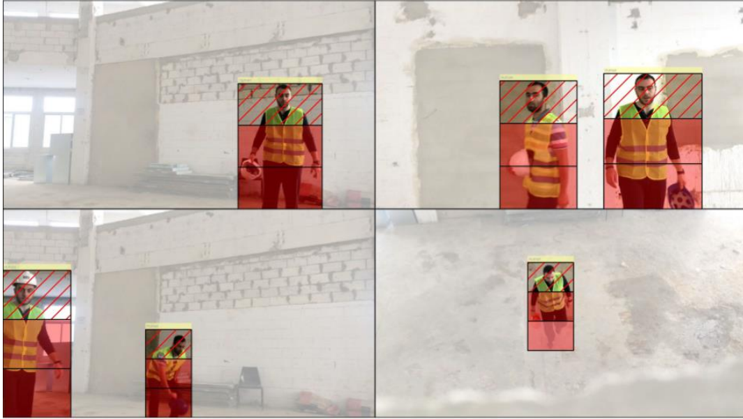
Figure 3.29: Hardhats not worn by workers – Outside the region of interest
