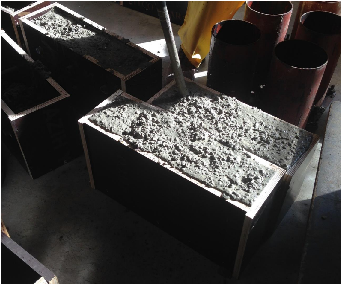
Figure AI-2 – Casting concrete in pre-pared molds
