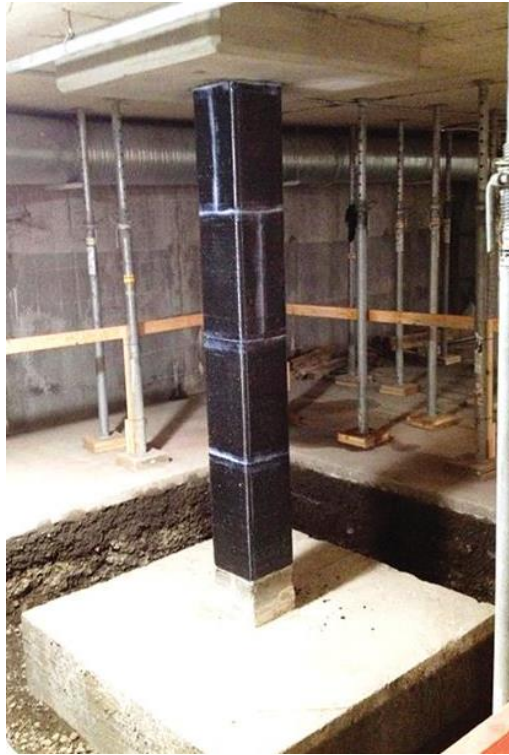
Figure I-1 - FRP-wrapped concrete column (Black, 2014)
