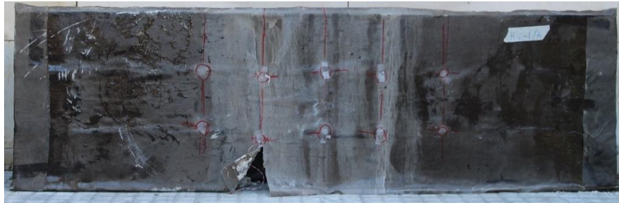
Figure 4.25 Failure Mode of H2-b (vertical view).
