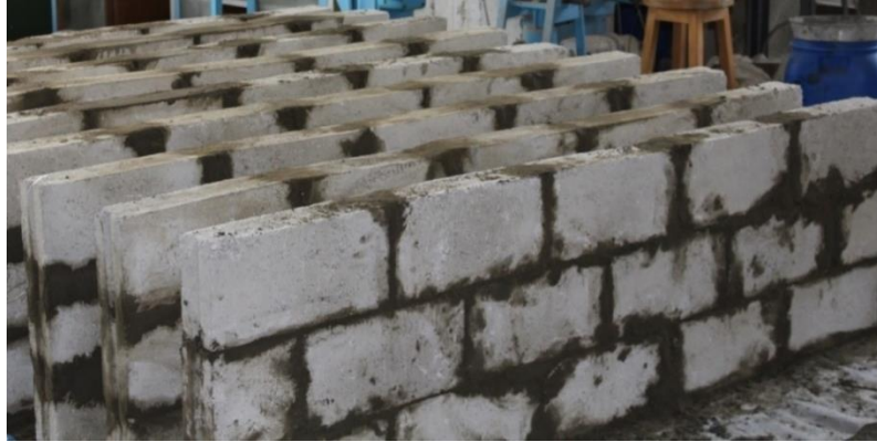
Figure 3.19 Fully Constructed Masonry Walls.
