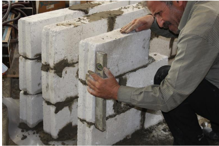
Figure 3.18 Mason Leveling the Walls.
