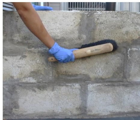
Figure 3.20 Surface Preparation for Hemp Fiber Fabric Installation.
