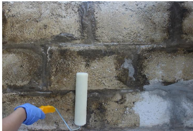
Figure 3.22 Application of Primer prior to Hemp Fiber Fabric Installation.
