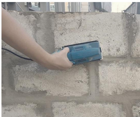
Figure 3.20 Surface Preparation for Hemp Fiber Fabric Installation.
