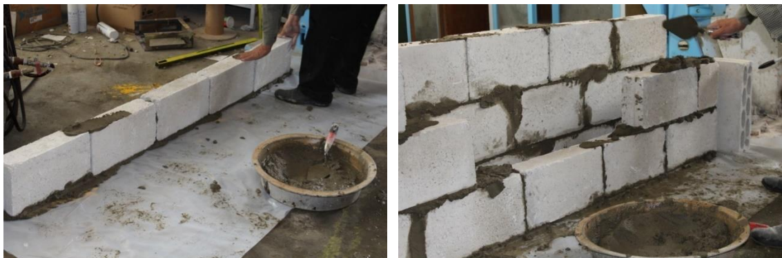
Figure 3.17 Mason Laying First and Second Course of CMU.
