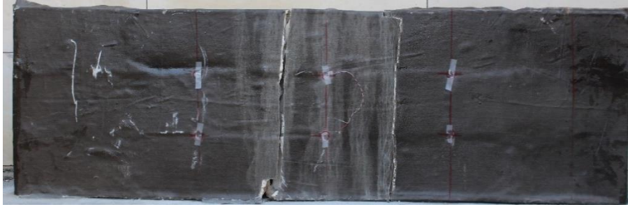
Figure 4.21 Failure Mode of H1-b (vertical view).
