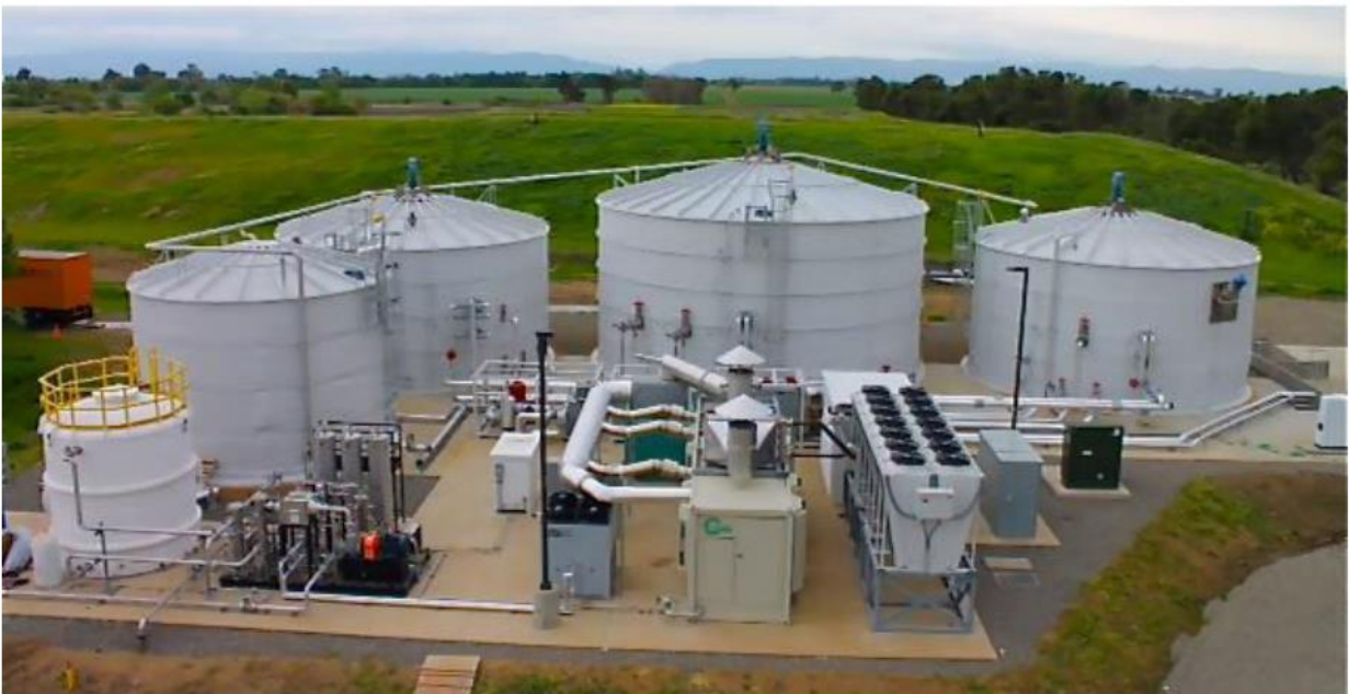
Figure 11: Renewable Energy Anaerobic Digestion Facility – UC Davis Biodigester (Zhang, 2015)
