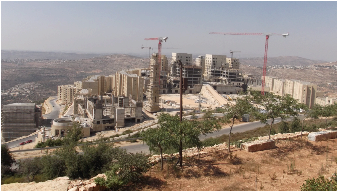
FIGURE 6. Rawabi construction site, July 2015 ( Photo by Author ).
