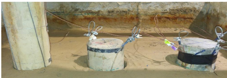
Figure 13. Piles installation procedure
