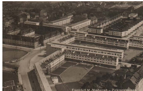
Figure 12: Siedlung Zickzackhausen by Ernst May, Frankfurt, 1926, Source: Pinterest
