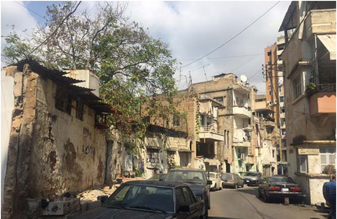
Figure 100: Inner Road in Al-Tamlis (Before)
