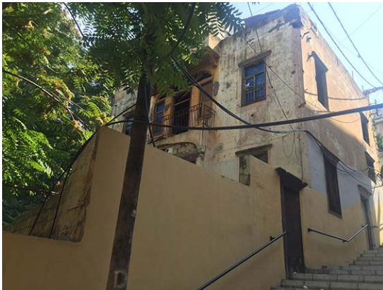
Figure 92: Heritage Building on Tamlis Staircase
