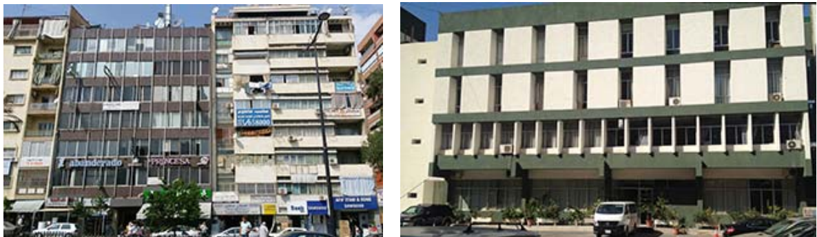
Figure 72: Barbour's Corniche Front (Left) and Maqassed Complex (Right)
