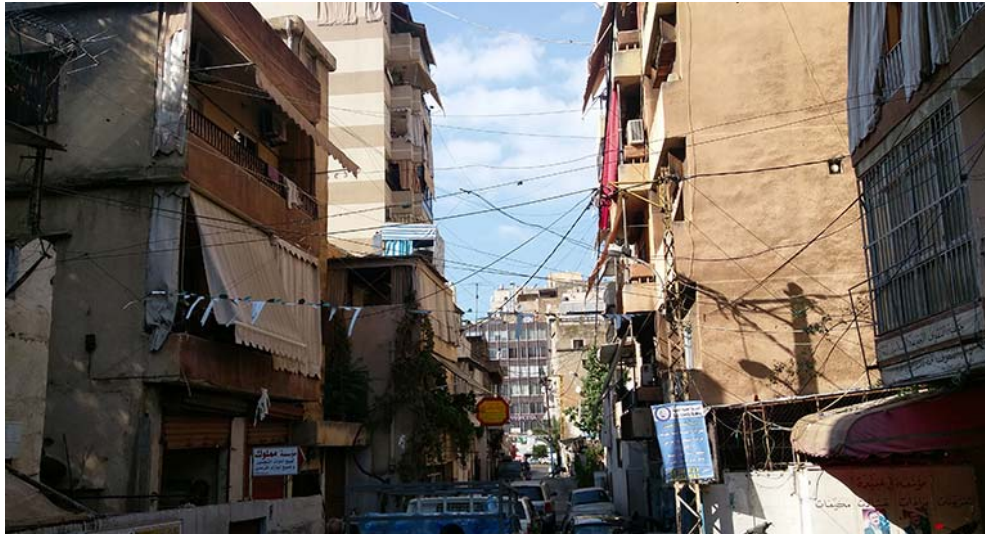
Figure 78: Al-Tamlis Road (Before)
