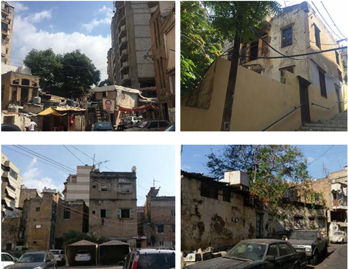
Figure 66: Run-down dilapidated blocks of housing (few historic) are a ubiquitous feature in the scenery of al-Tamlis
