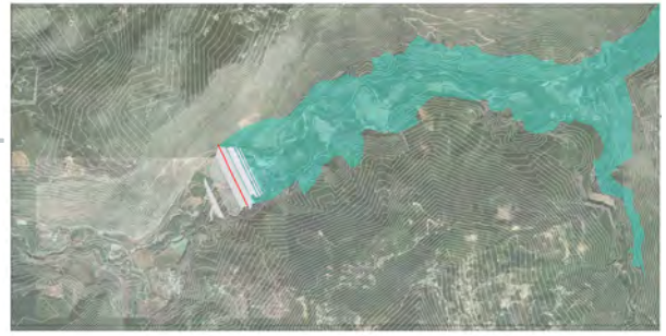
The Dam Area
