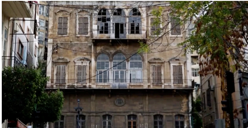
Picture 8 – The façade of the Boustani house in 2018
