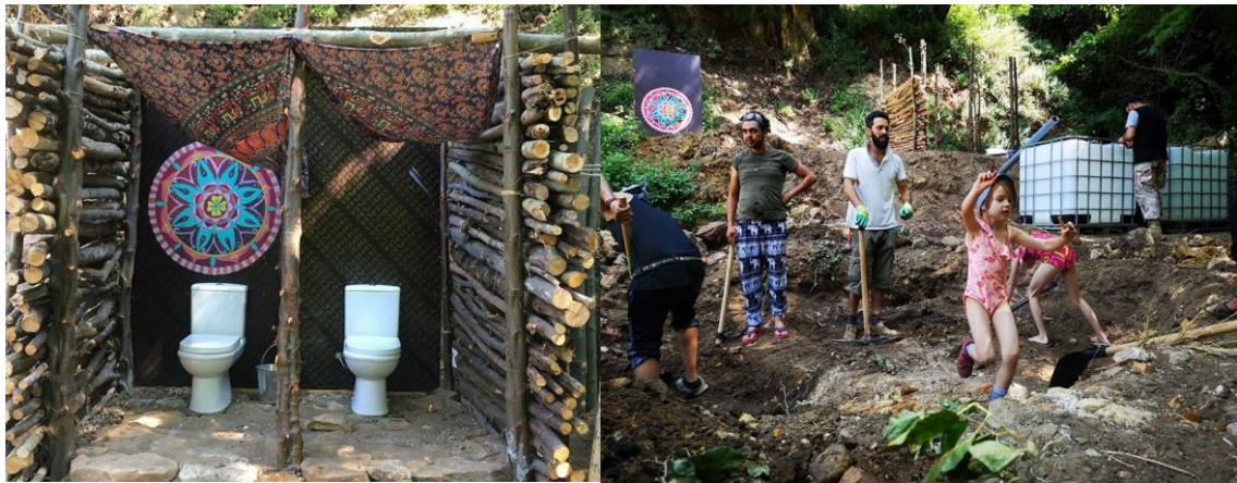
Figure 17: DIY vermicomposting sewerage system based on a flush toilet in Chouf, Lebanon (Source: LiPattern)
