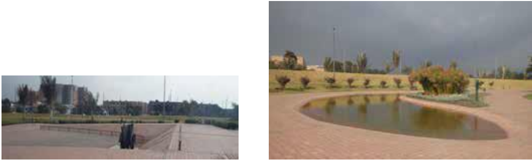
Figure 18: Different solutions for handling and displaying run-off water in Public place in the park at library Virgilio Barco, Bogota.
