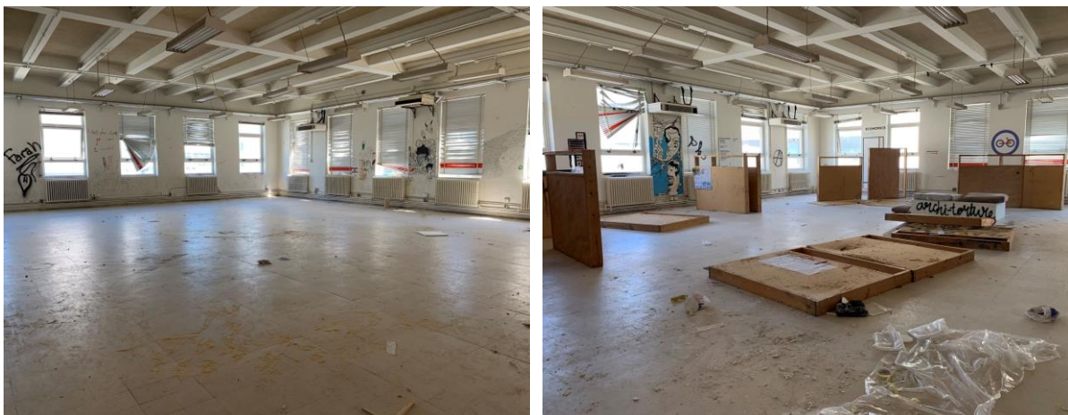
Figure 4 – Example of Architecture Classrooms (During Renovation)
