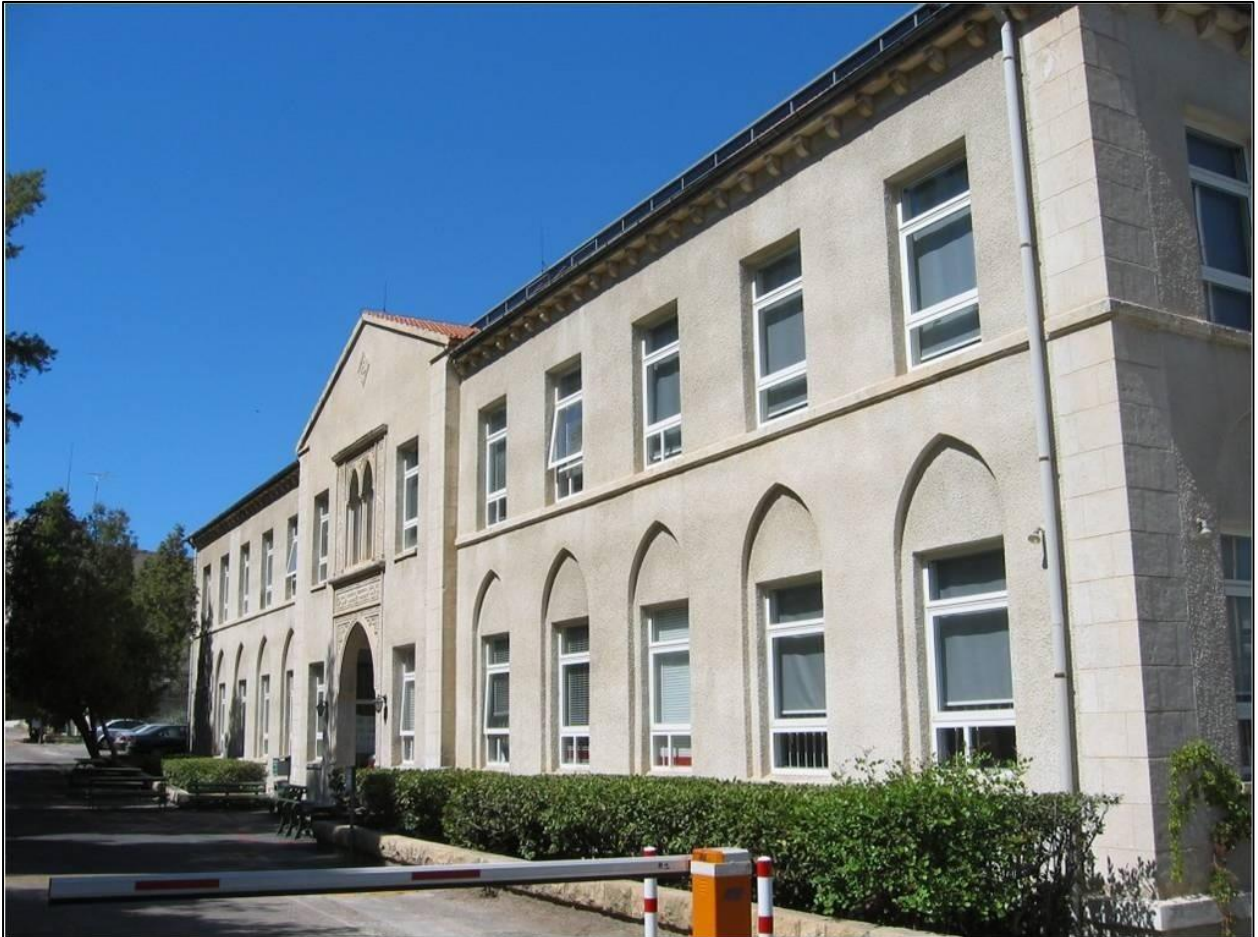
Figure 7 – Dar Al-Handasah Architecture building
