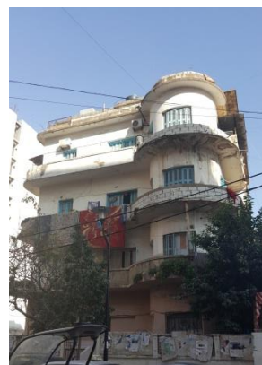
Figure 3: Evicted building to be demolished in TJ (2018)
