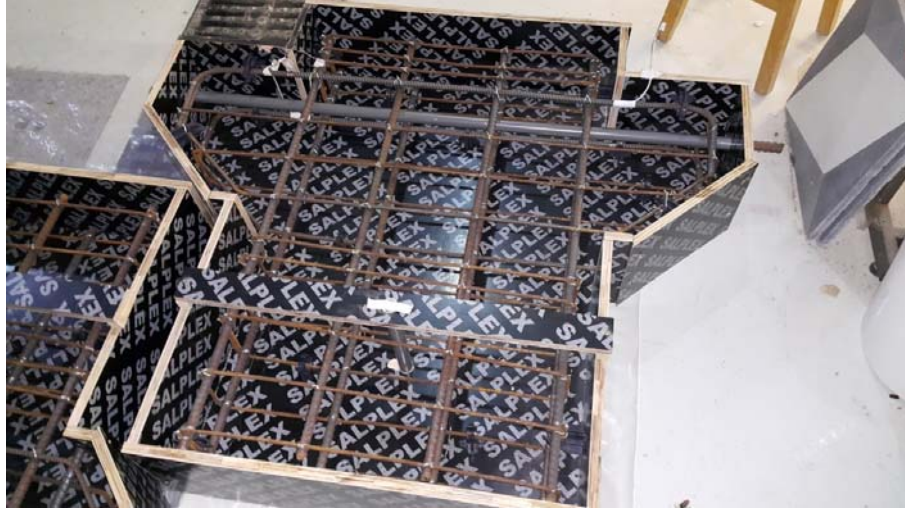
Fig. 5. S1-1B before casting
