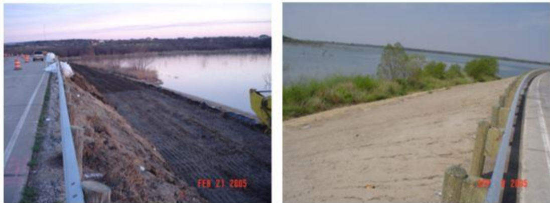
Figure 1.5 Lake Ridge parkway slope repair project (from Gregory, 2006)
