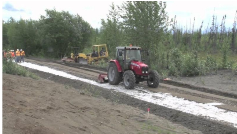
Figure 1.3 Conventional tractor and roller compactor used for field placement of fibers (from YouTube, UAF College of Engineering & Mines, 2010)
