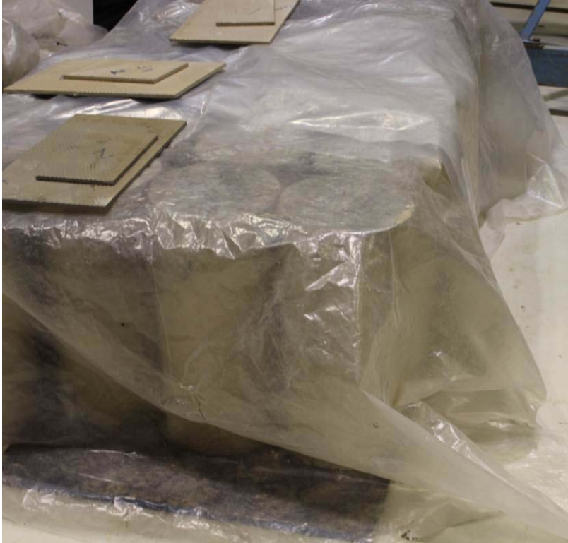
Figure 27 Curing of concrete columns
