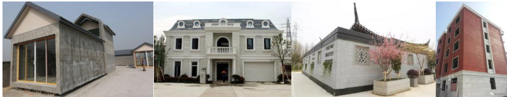
Figure 6. Winsun 3D printed project samples. (1) Ten printed houses, (2) 3D printed villa, (3) 3D printed courtyard, (4) 6 story 3D printed building.
