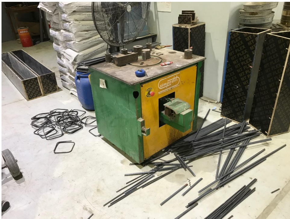
Figure 36. Fabrication of steel bars and stirrups
