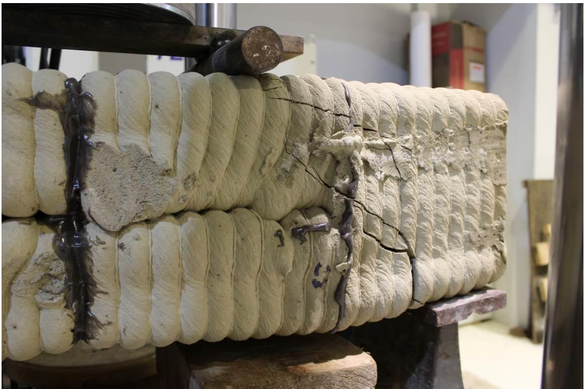
Figure 70. Cracked beam P:4-3
