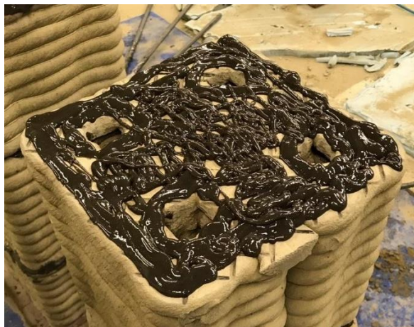
Figure 28. Application of Epoxy to the prepared concrete surface
