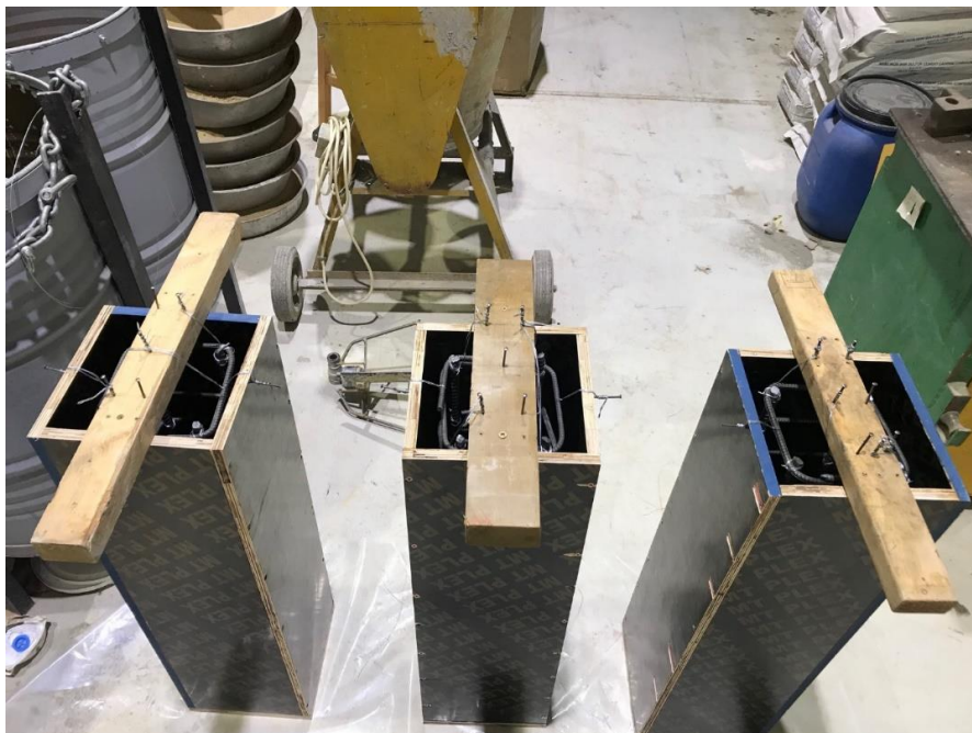
Figure 34. C:4 Samples ready for casting
