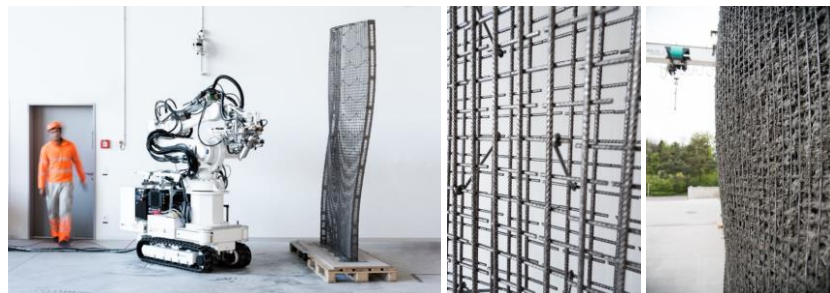
Figure 15. Mesh Mould reinforcement typology and concrete infill
