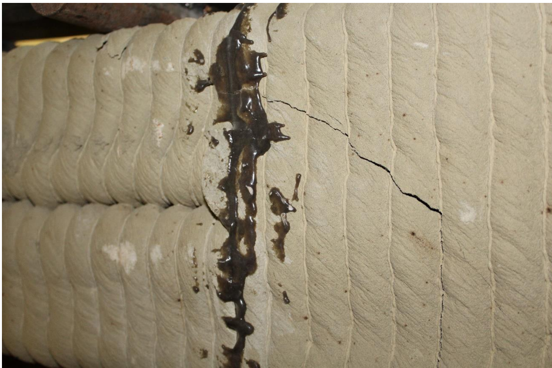
Figure 65. Diagonal crack propagating along the interface between two 3D printed filaments
