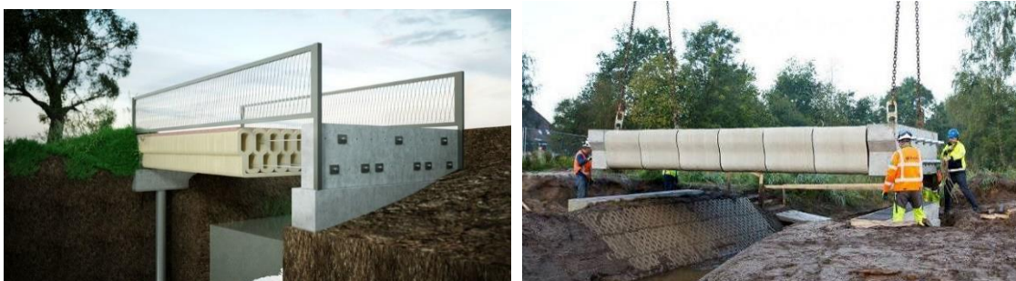
Figure 9. 3D printed Cyclist Bridge. (1) Cross section of the bridge showing pre-stressed strands, (2) assembling the 3D printed bridge on-site by BAM Infra
