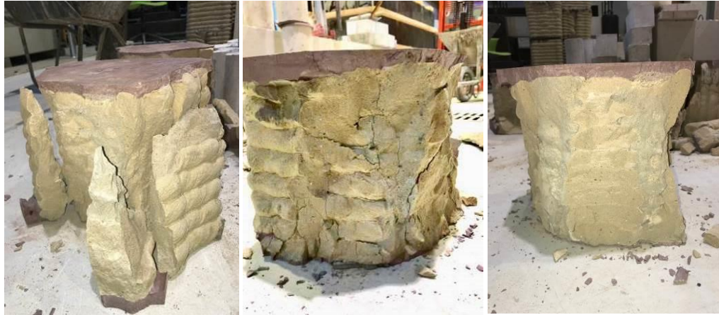
Figure 52. Concrete edge spalling and fracture plane in PH:1 samples
