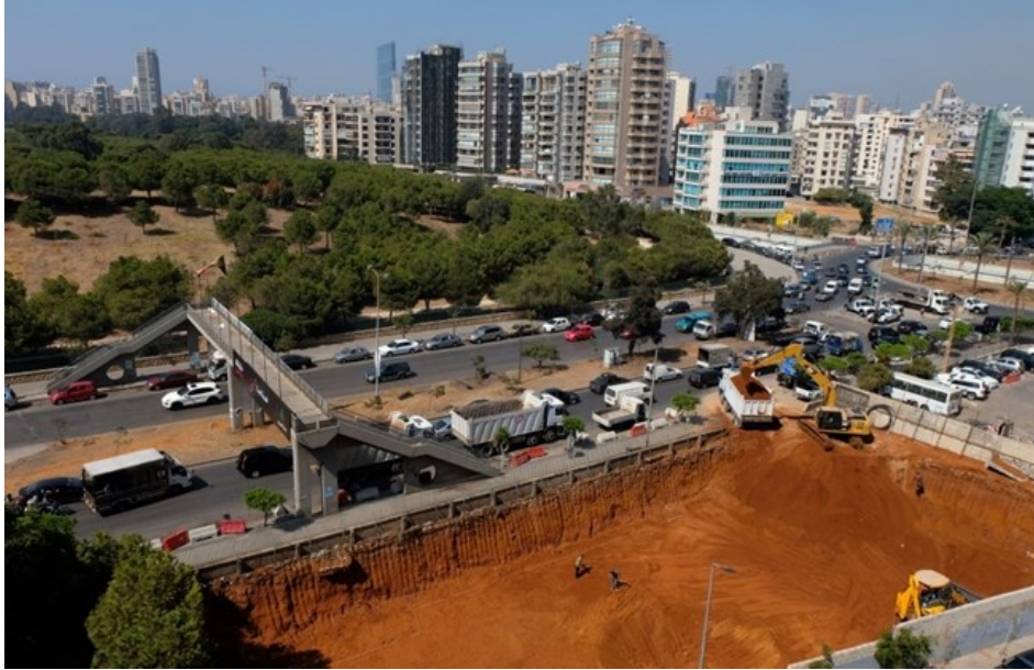
Figure 54. Excavation at Horsh Beirut (Source: The Daily Star Lebanon,2018)
