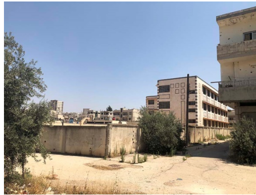
Figure 83: Intact buildings ( Source: the author )
