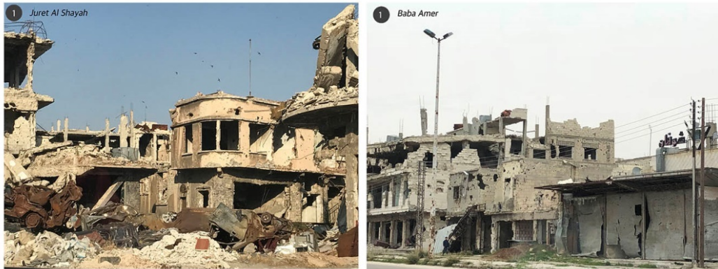
Figure 65: Heavily damaged neighborhoods ( Source: the author ).
