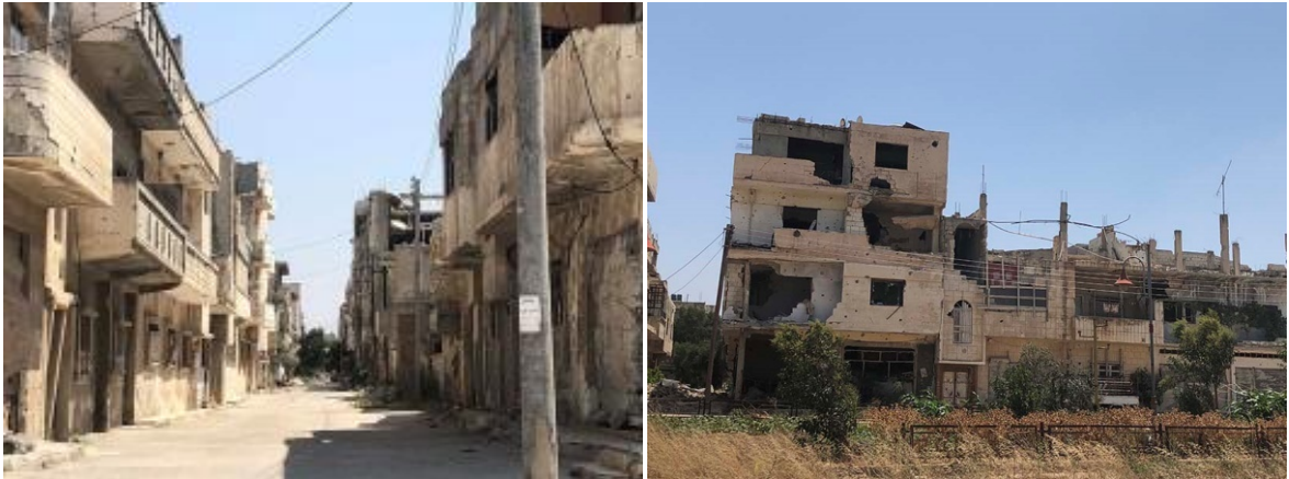
Figure 81: Medium levels of damage ( Source: the author )
