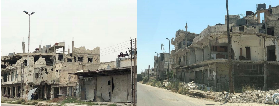
Figure 80: High levels of damage ( Source: the author )
