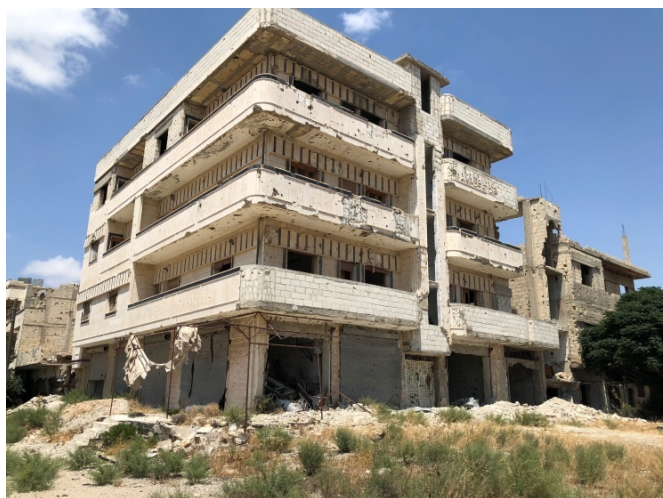
Figure 48: New buildings in Baba Amer ( Source: the author ).
