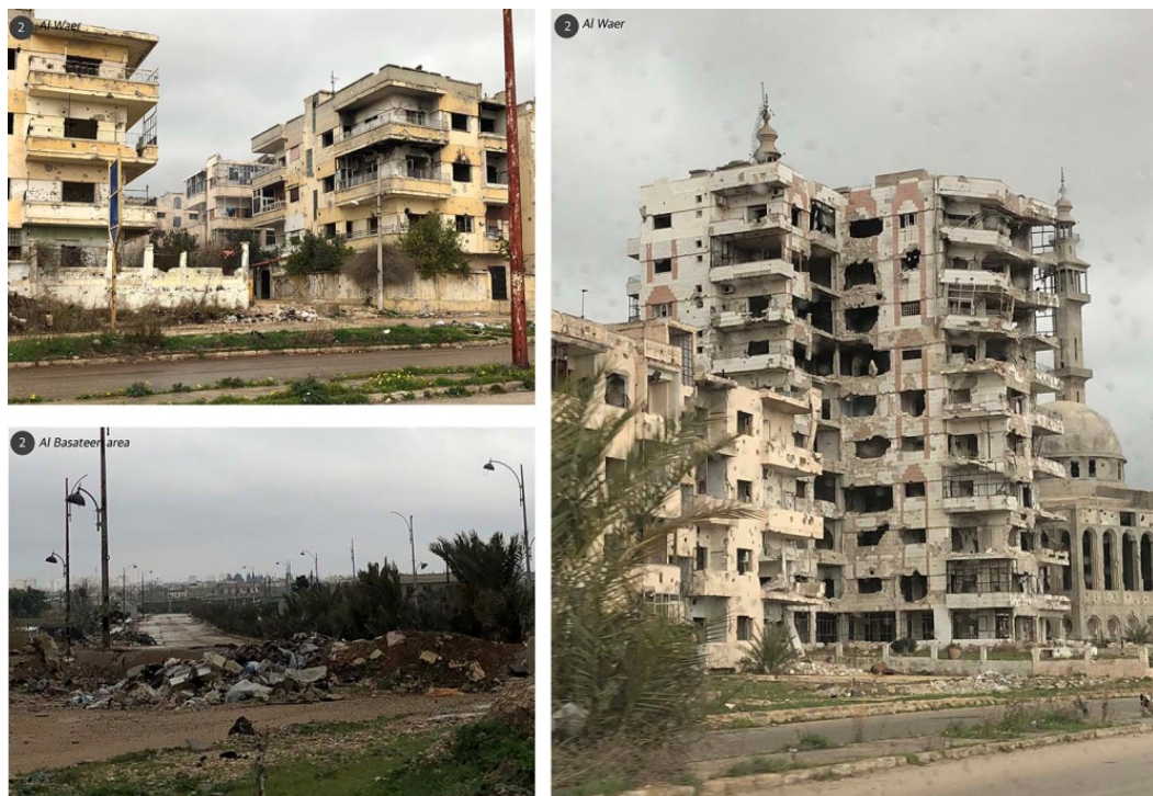
Figure 66: Partially damaged neighborhoods ( Source: the author ).
