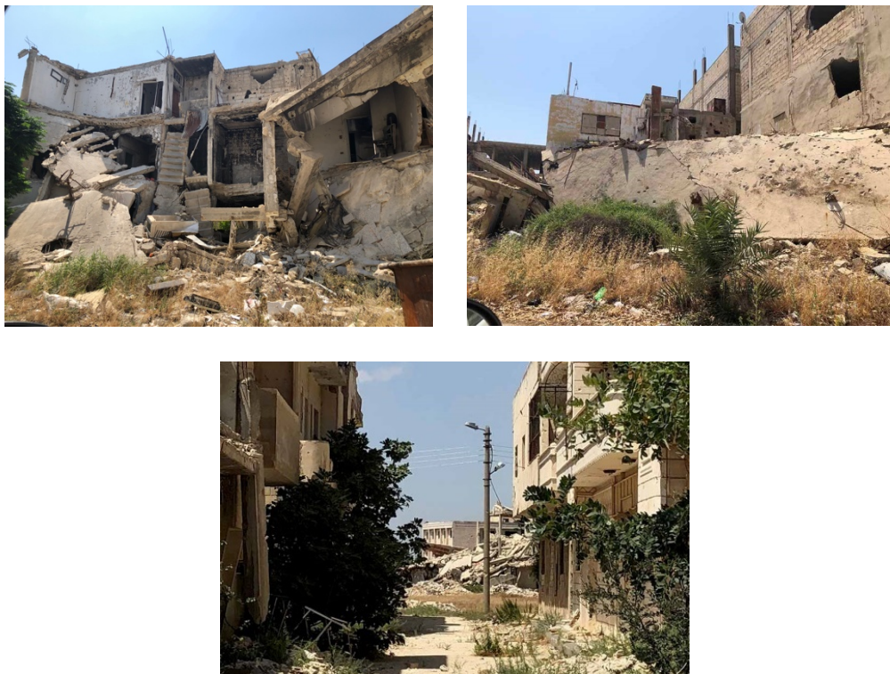
Figure 77: Completely destroyed buildings ( Source: the author ).
