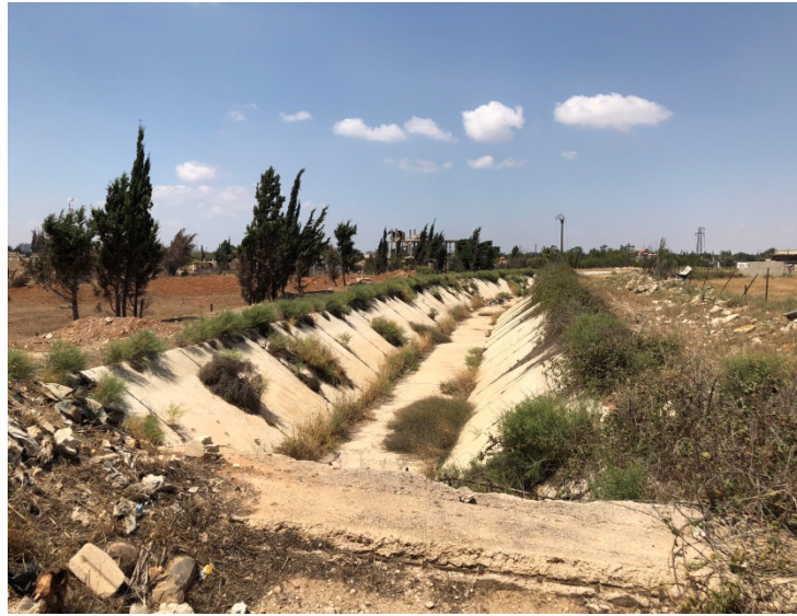
Figure 50: Baba Amer irrigation canal ( Source: the author ).
