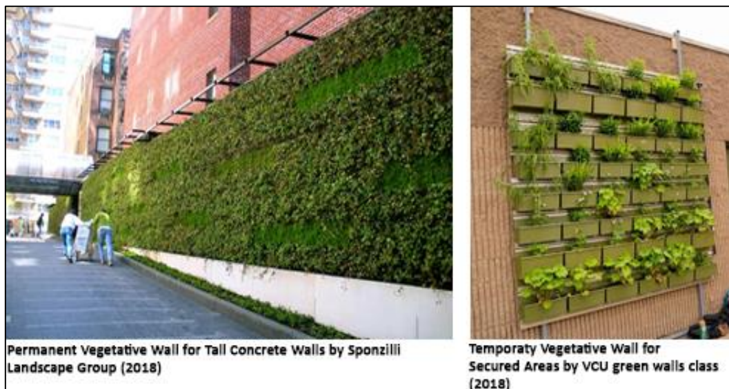
Figure 85: [Examples of Vertical Landscape Infrastructure for Permanent and Temporary Usage], Al Asmar 2018
