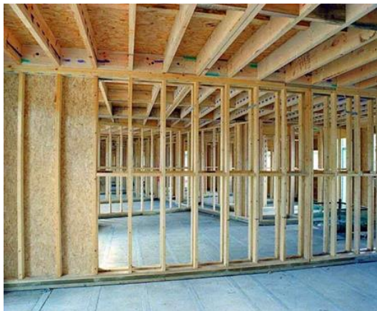
Figure 14 – Open panel timber frames (Hashemi et al., 2016)
