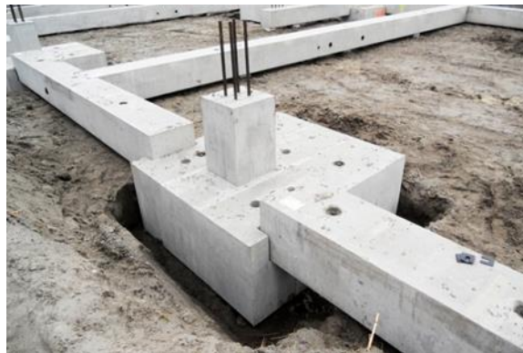
Figure 7 – Precast concrete foundations (Hashemi et al., 2016)
