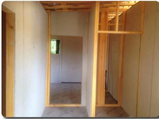
Figure 15 – Closed panel timber frames (Hashemi et al., 2016)
