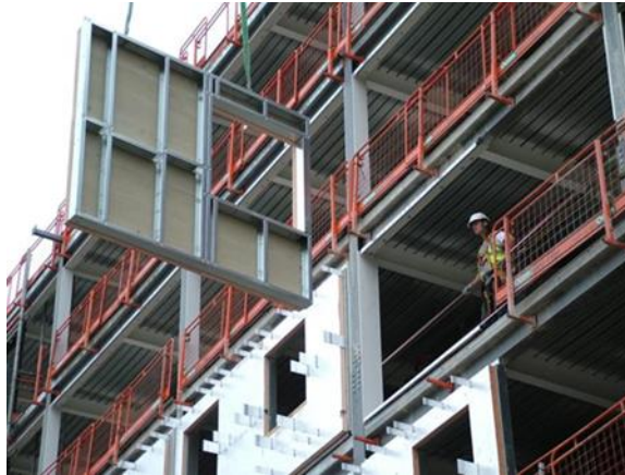
Figure 10 –Lightweight steel closed panels (Hashemi et al., 2016)
