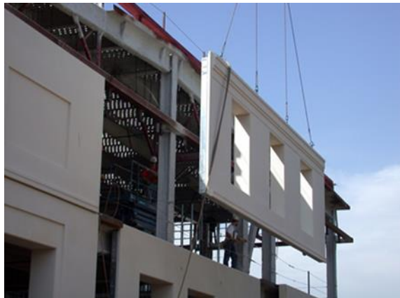
Figure 11 –Precast concrete panels (Hashemi et al., 2016)
