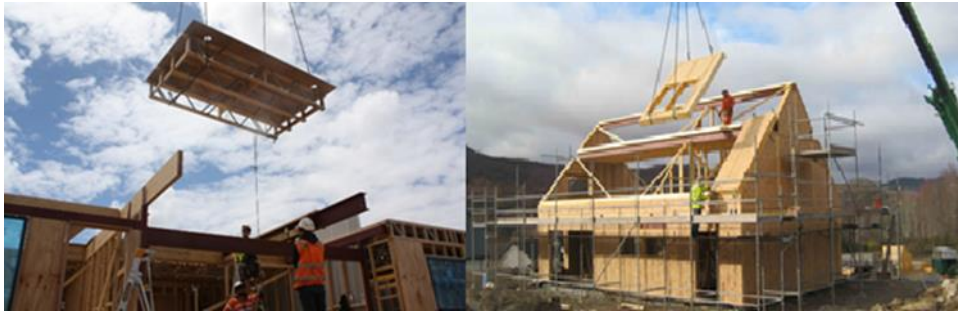
Figure 8 –Floor and roof cassettes (Hashemi et al., 2016)
