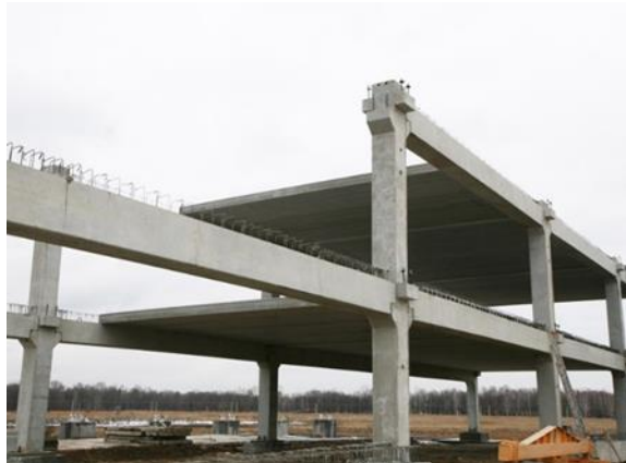
Figure 5 – Precast concrete frames (Hashemi et al., 2016)
