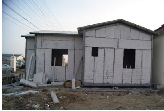
Figure 12 – Light-weight composite solid precast sandwich panels (Hashemi et al., 2016)
