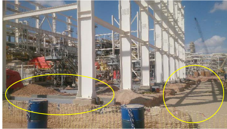
Figure 21 Trenches surrounding Unit 42 sunshade (Dec 2017)
