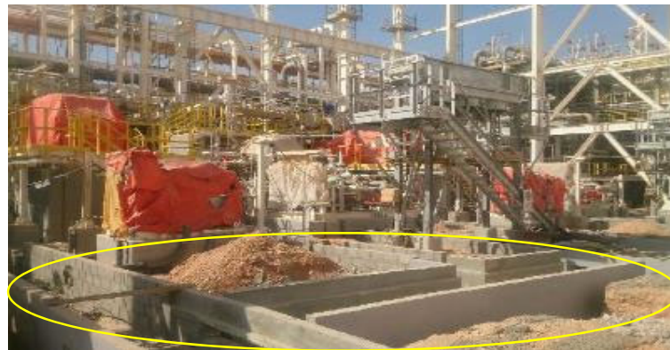
Figure 22 Trenches inside unit 42 (Dec 2017)
